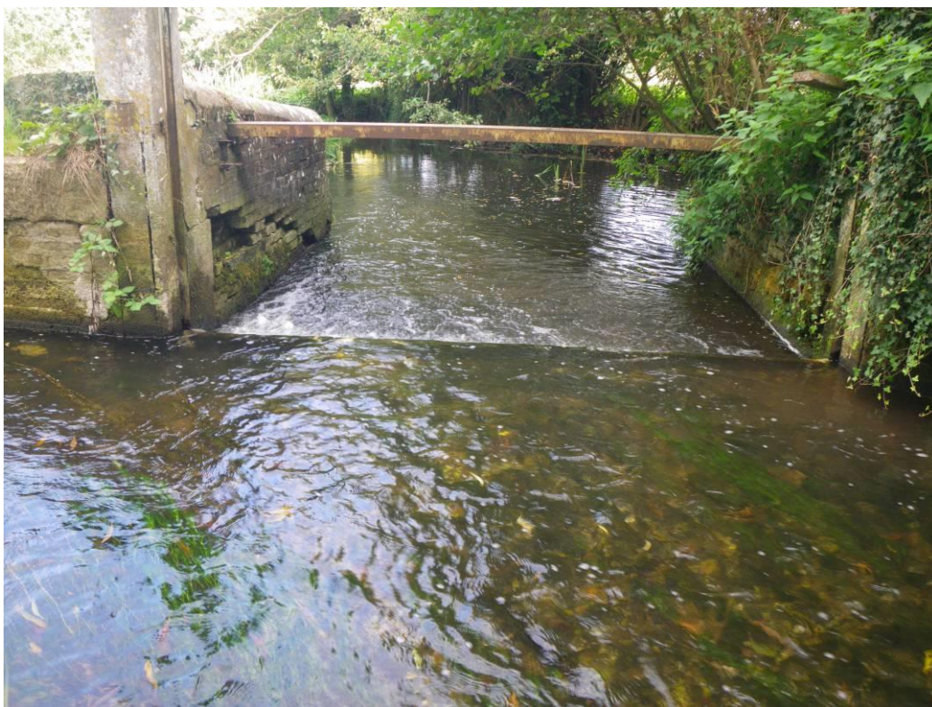
Photo 9. Derelict weir structure located near the bottom boundary.
