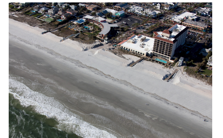
Completed Berm and Dune
