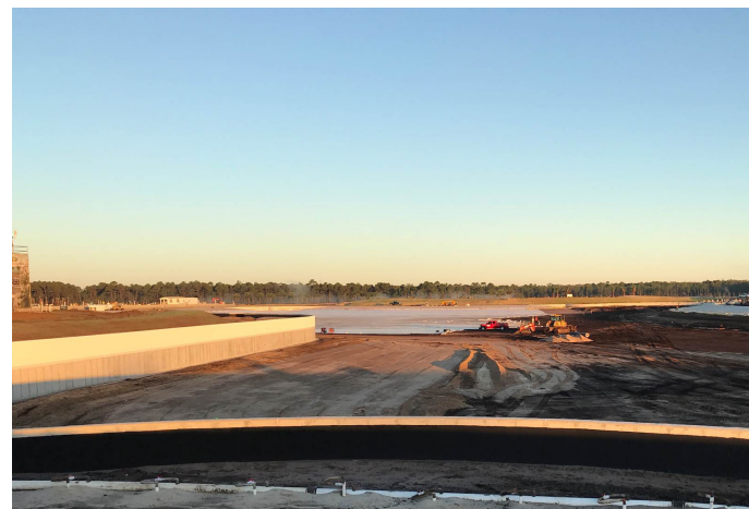
Water Filling the Lined Lagoon
