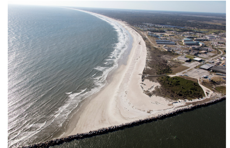
Completed Dune Restoration
