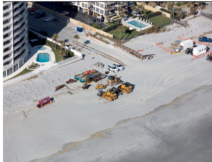
Berm and Dune Structure Construction
