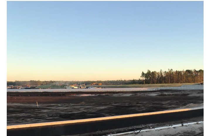
Cast-in-place Retaining Wall and Temporary Dewatering System Outside the Wall
