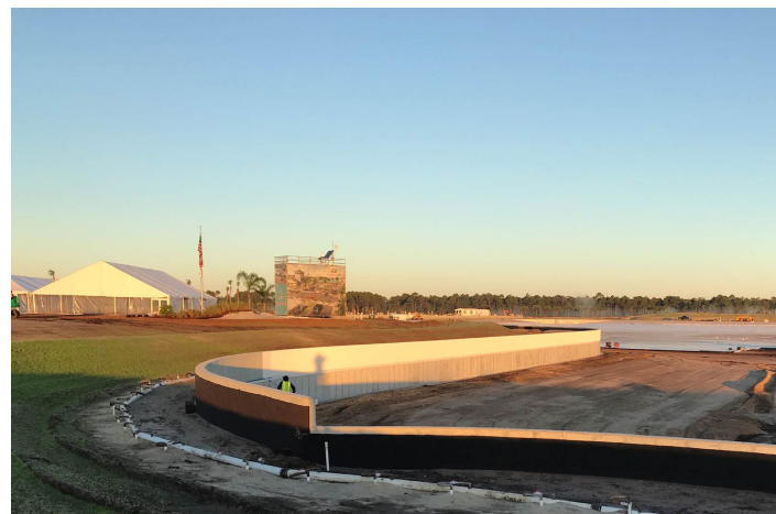
Retaining Wall, Temporary Dewatering System, Liner Placement, and Beach Liner
