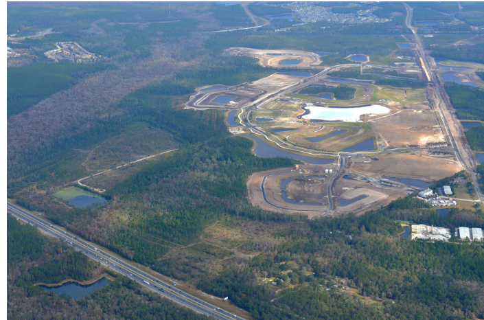
Aerial of Development and Lagoon with Completed Liner
