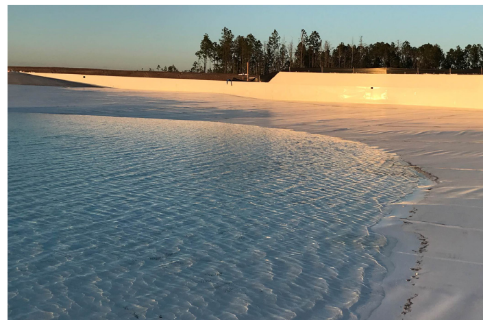
Retaining Wall, Temporary Dewatering System, and Beach Liner
