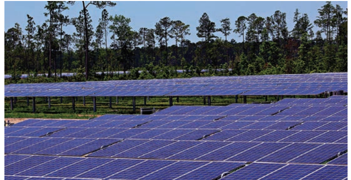
The Montgomery Solar Project is the Newest Solar Photovoltaic Project to come on-line in JEA's Service Territory
