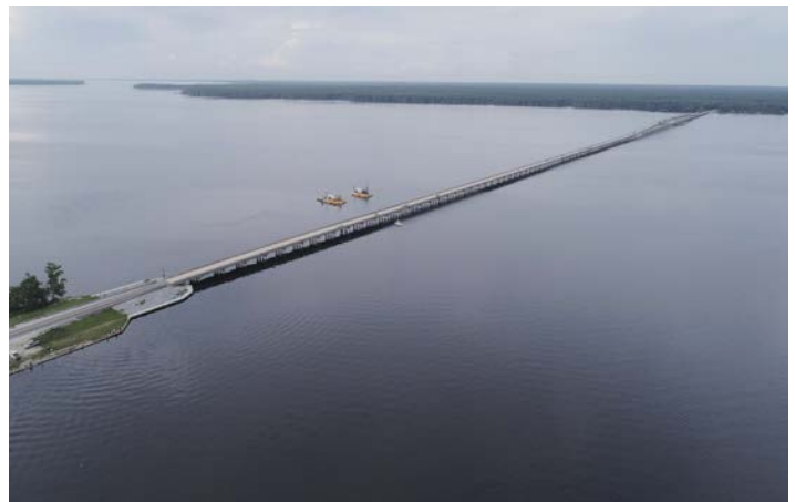
Expanded view of Terracon drill rigs drilling on barges for the Shands Bridge Replacement job in St John's County, Fla.
