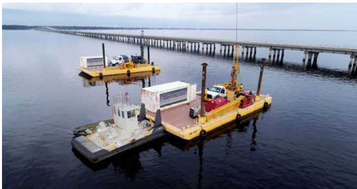
Terracon Drill Rigs Drilling on Barges for the Shands Bridge over St. John's River
