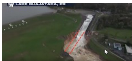
Figure 3. Red Lines Indicate Pre-hurricane Outline of the Spillway Chute Invert
