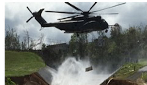
Figure 4. CH 53 Helicopter Dropping a Concrete Jersey Barrier
