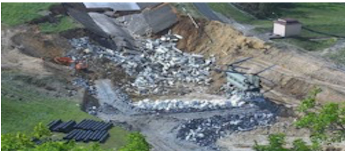
Figure 5. Jersey Barriers and Large Sand Bags Forming a Stilling Basin
