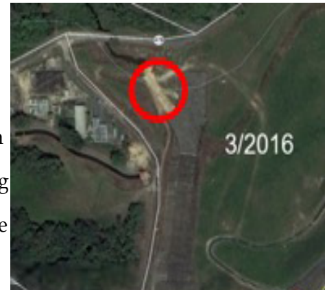
Figure 6. Aerial View of Erosion of the Northwest (left) Side of the Spillway Near the Discharge End Following Spillway Releases in November 2015 and March 2016
