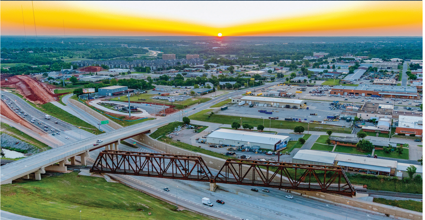
I-235 Broadway I-44 Interchange Oklahoma City, OK Engineering by Haskell
