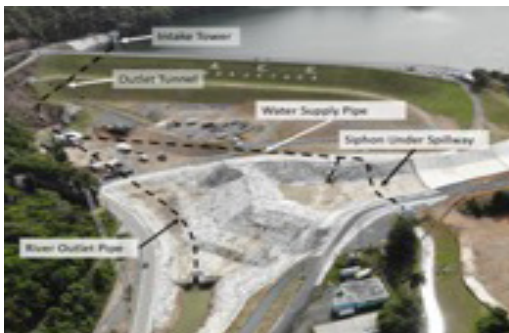
Figure 7. Aerial of Repaired Spillway
