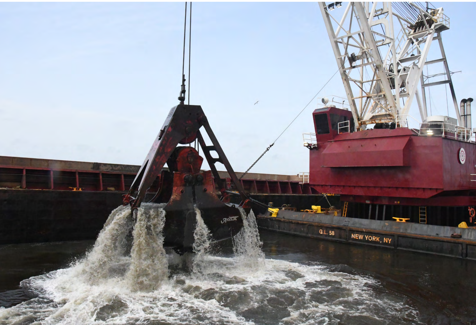
A clamshell dredger removes a batch from the river bed during a ribbon cutting ceremony that marked the completion of the Harbor Deepening Project at the Blount Island Marine Terminal Monday, May 23, 2022 at JaxPort in Jacksonville, FL. (USACE photo by Mark Rankin)
