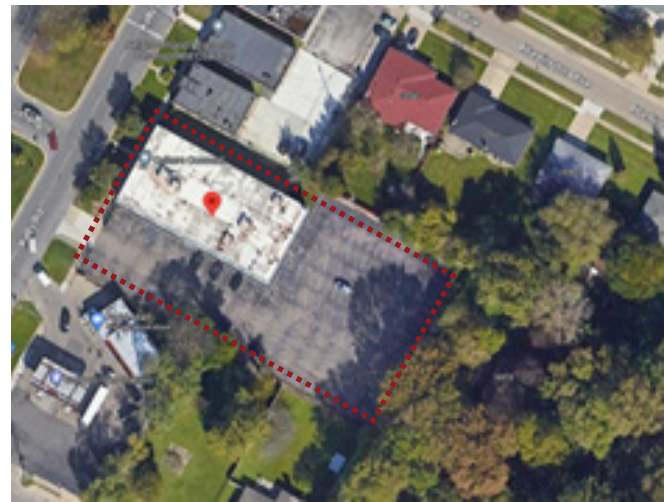
Current condition of 19992 Kelly
