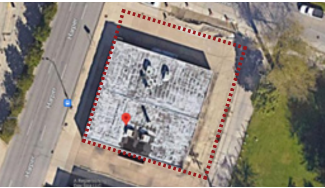
Current condition of 20790 Harper
