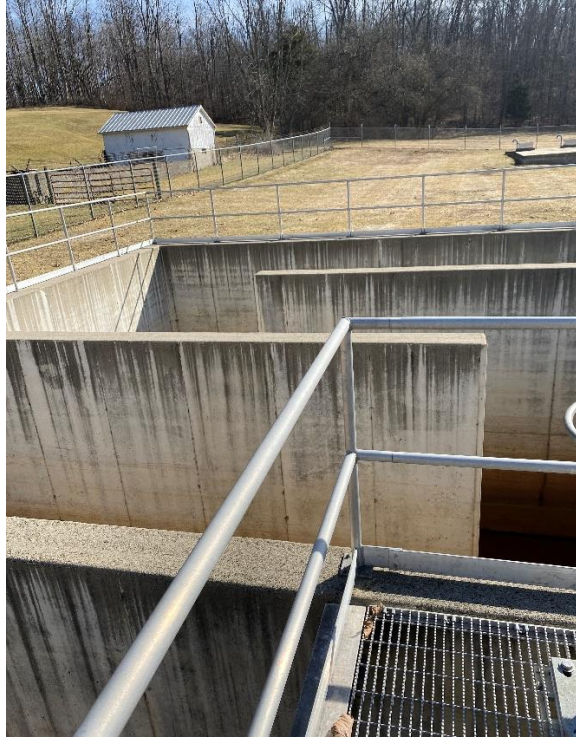
WTP – Cast-in-Place Concrete Backwash EQ Basin
