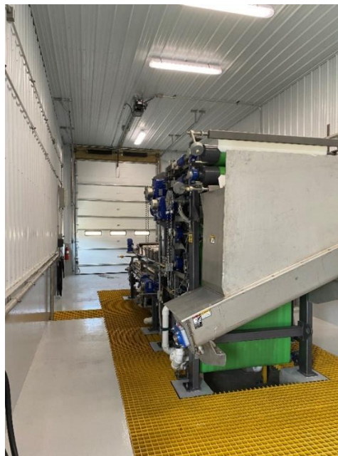
Lakengren WWTW ~ Sludge Belt Press (in Sludge Press Building)
