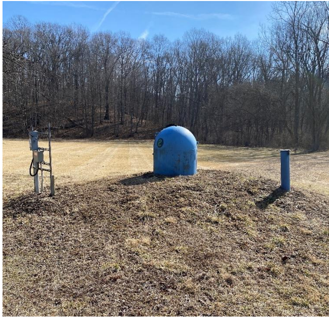
Well #3 - Lakengren Water Treatment Facility (note well #2 casing was reused, thus marked #2)
