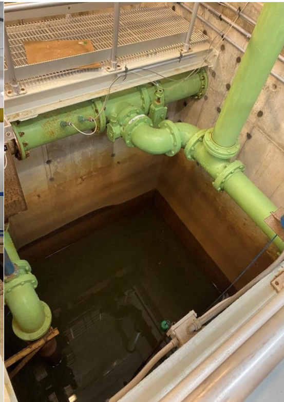
WTP – Cast-in-Place Concrete Gravity Iron filter
