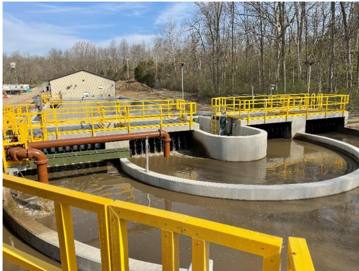
Lakengren WWTP ~ Surface Aerator Oxidation Ditches
