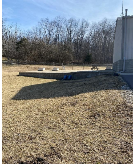
WTP – Post Filtration Clearwell
