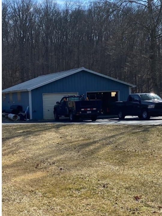
WTP – Maintenance Shop #1 (East)
