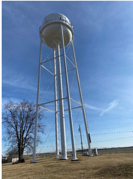
East Elevated Water Storage Tank – 200,000 gallons
