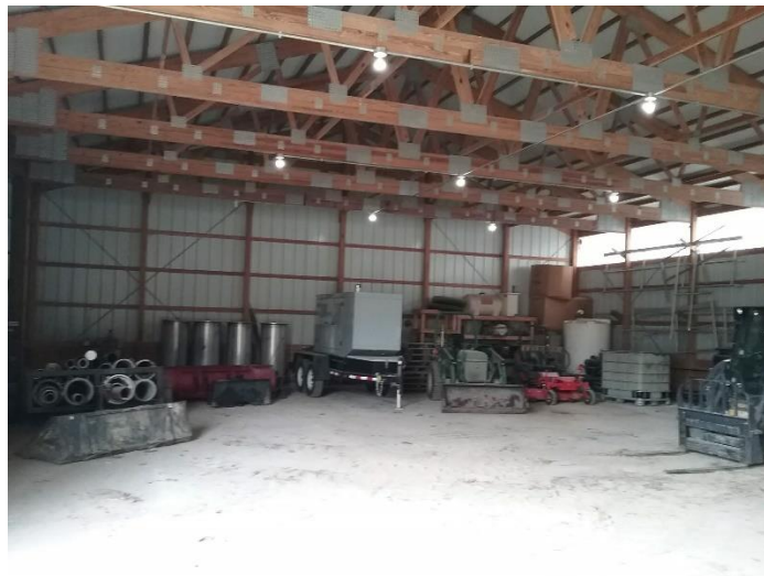
Lakengren WWTP ~ Maintenance Building
