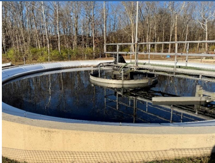
Lakengren WWTW ~ Secondary Clarifier #2
