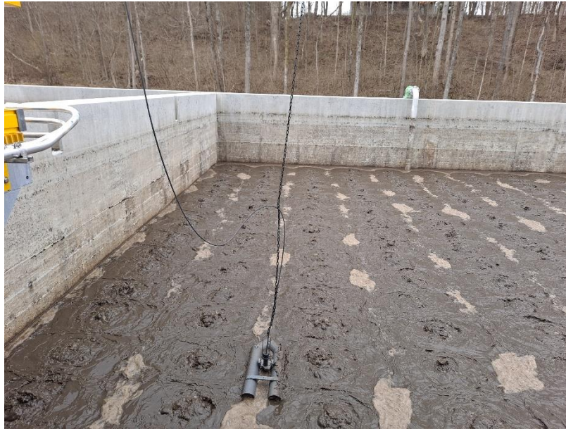
Lakengren WWTP ~ Sludge Digester Tank
