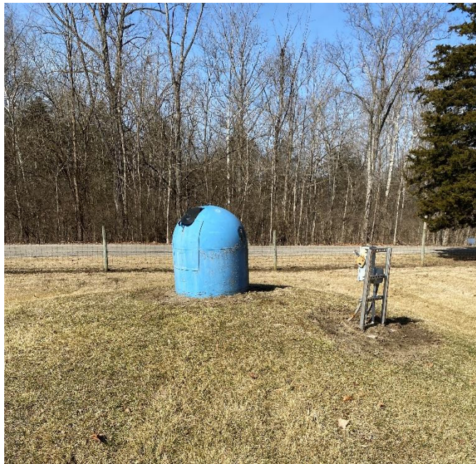
Well #1 - Lakengren Water Treatment Facility
