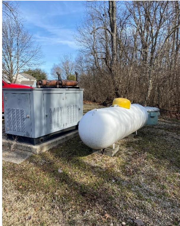
Sanitary Lift Station #3 –Fiberglass drywell (green, right) with generator & propane on left
