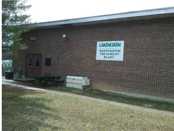
Lakengren WWTP ~ Lab Building
