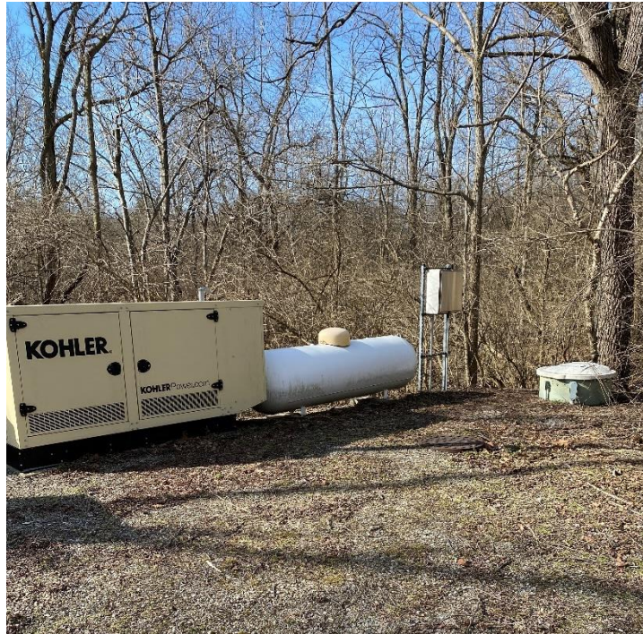
Sanitary Lift Station #4 –Fiberglass drywell (green, right) with generator & propane on left
