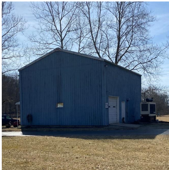
WTP – Maintenance Shop #2 (East)
