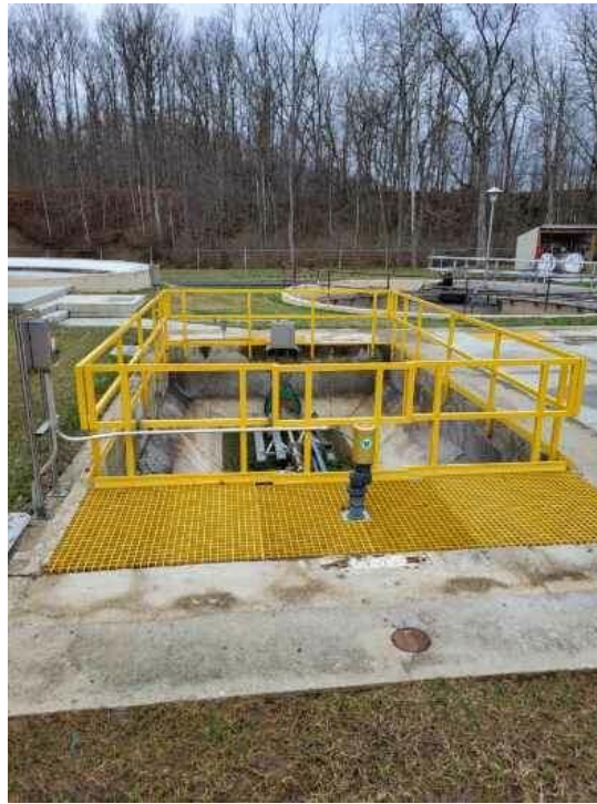
Lakengren WWTP ~ Flocculator & Rapid Mix Tank
