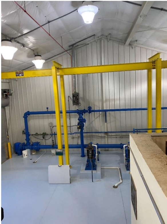
WTP – High Service Pumps & Piping
