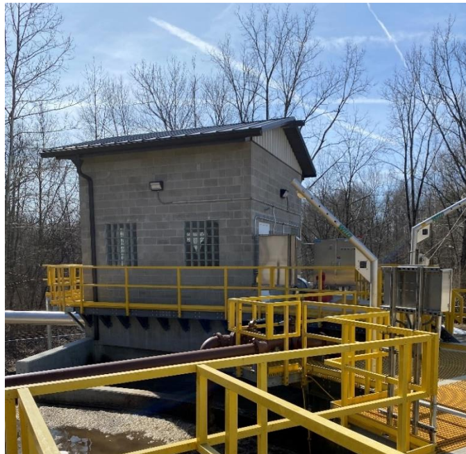
Lakengren WWTP ~ Influent Screening/Grit Removal Building
