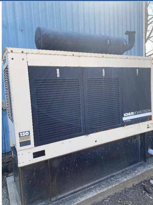
WTP - Kohler 150kW Diesel Generator
