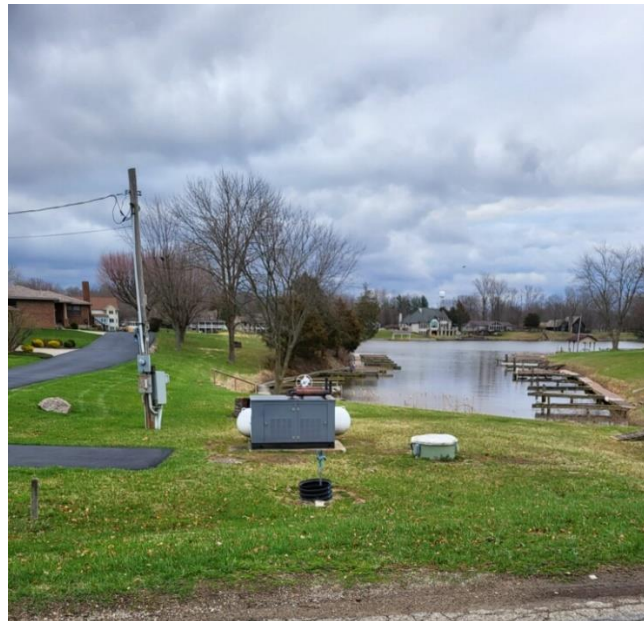
Sanitary Lift Station #1 –Fiberglass drywell (green, right) with generator (left) & propane tank behind
