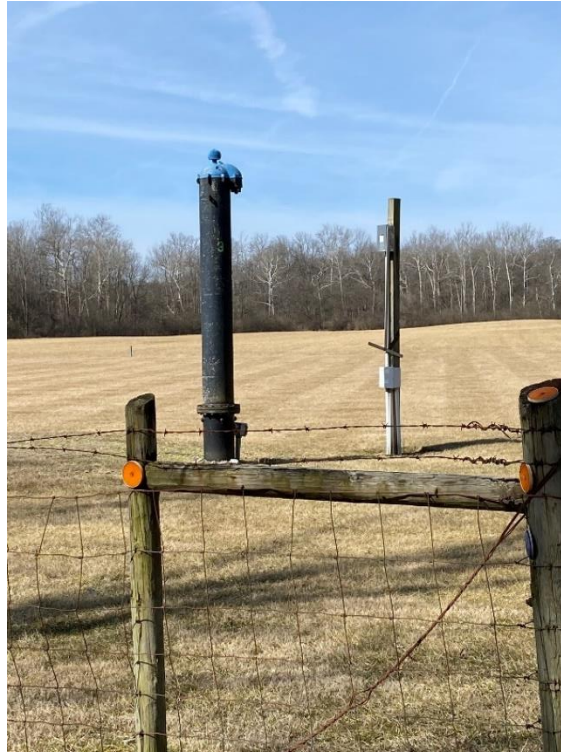
Well #4 - Lakengren Water Treatment Facility
