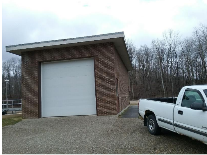
Lakengren WWTP ~ Shop Building
