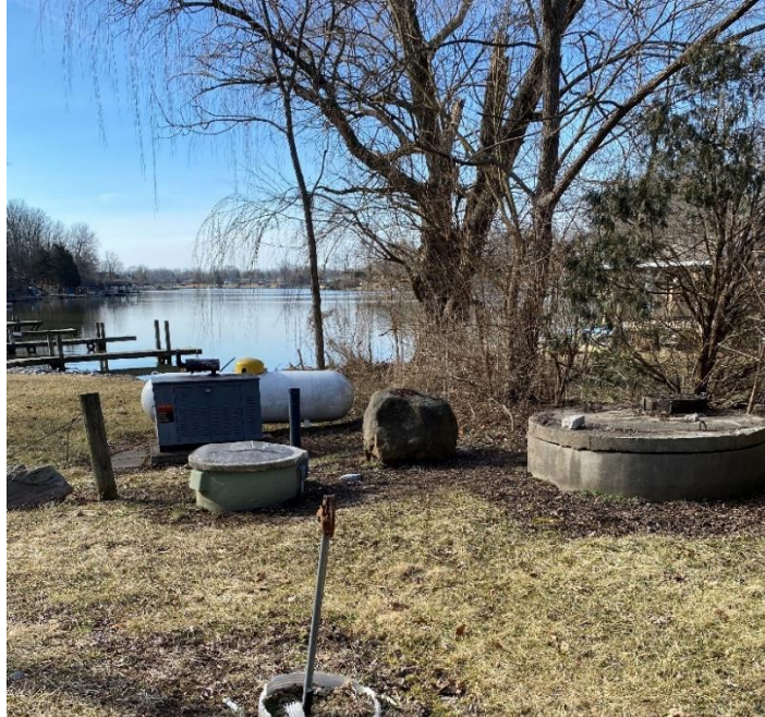
Sanitary Lift Station #2 – Precast Concrete Wetwell (right), fiberglass drywell (green, left) with generator & propane tank behind
