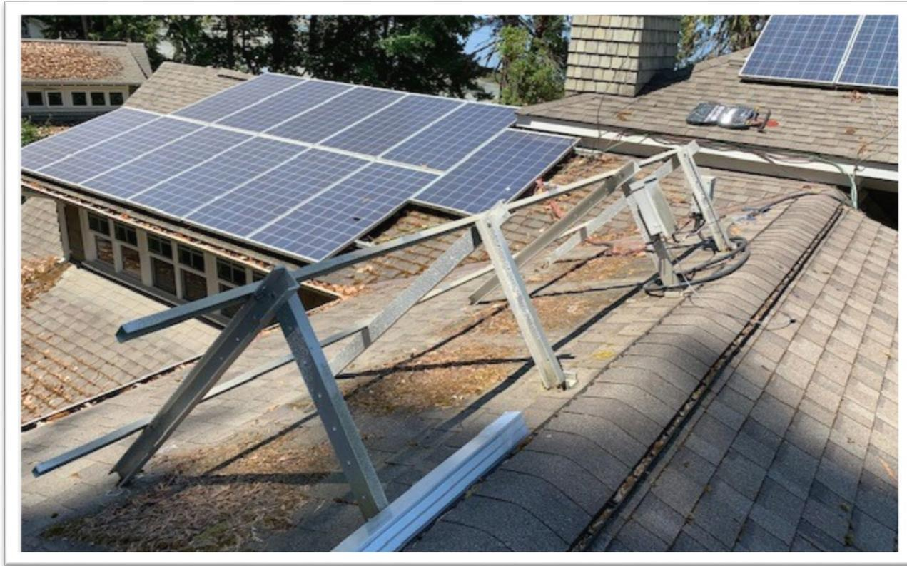
Re-built Panel frame at 80% degree angle with new supports using Fast-rack system to accommodate new 72 Cell Panels
