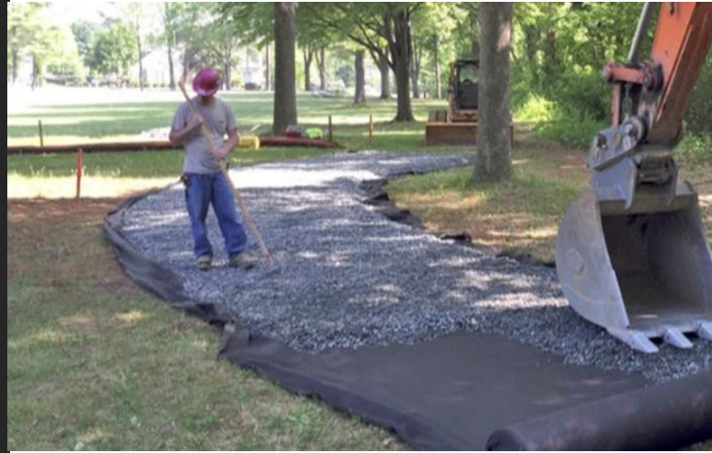
PLACE GEOTECH FABRIC AND STONE BASE
