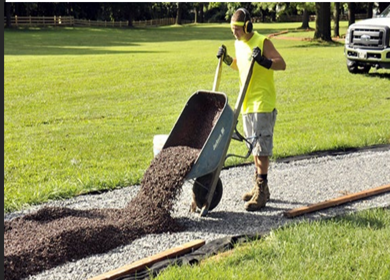
TRANSFER MIX TO POINT OF INSTALLATION
