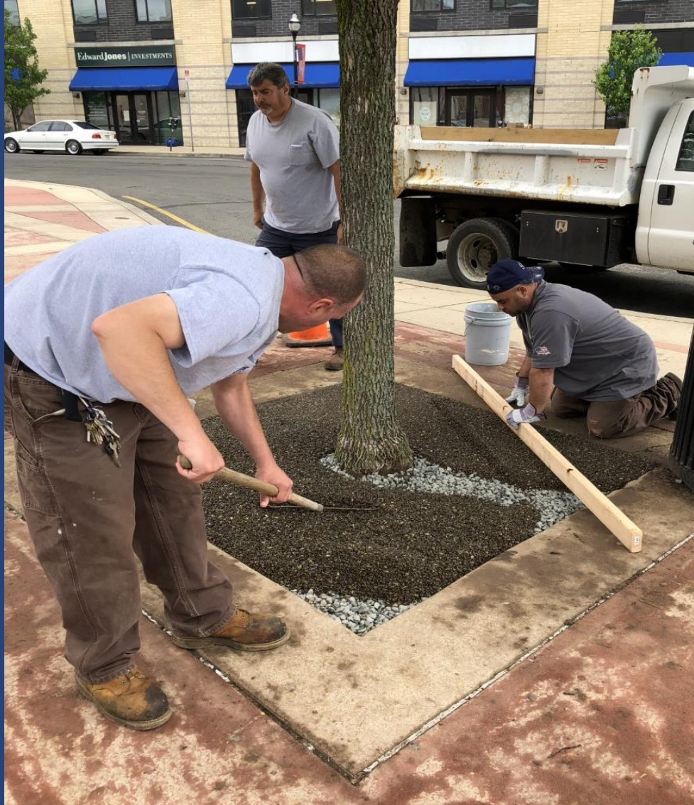
Pour, rake and screed material.
