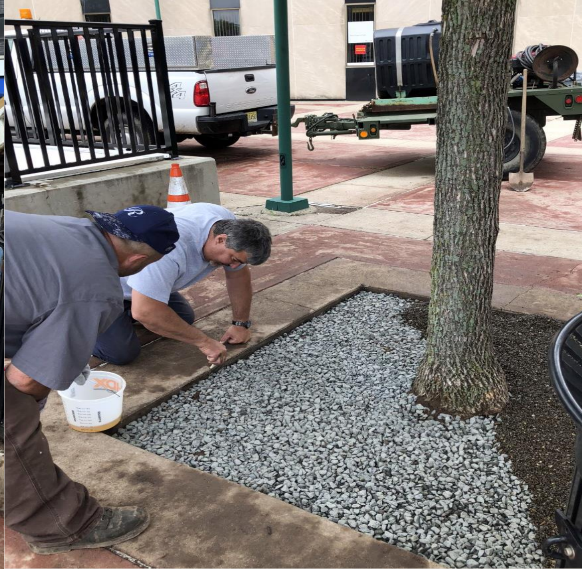
Coat edge of mating surfaces with binder. Note: Binder Stains
