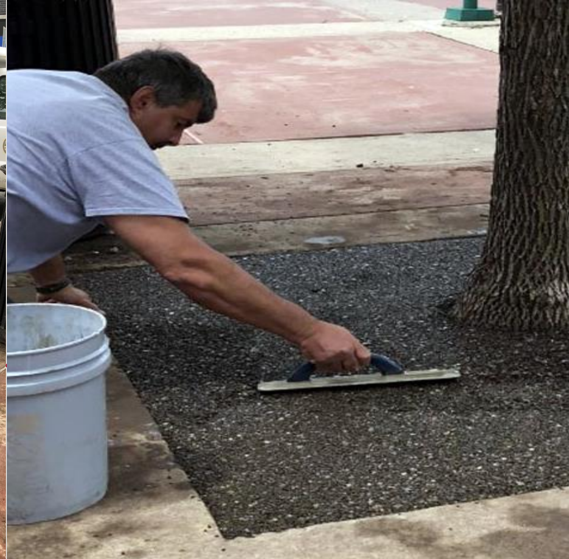
Finish surface with Mag float coated with cooking oil
