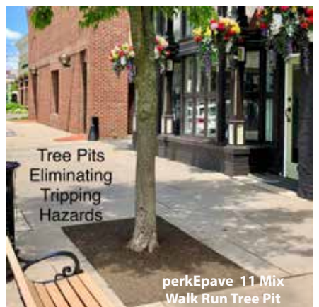
perkEpave tree boxes provide a clean and neat appearance and eliminates tripping hazards
