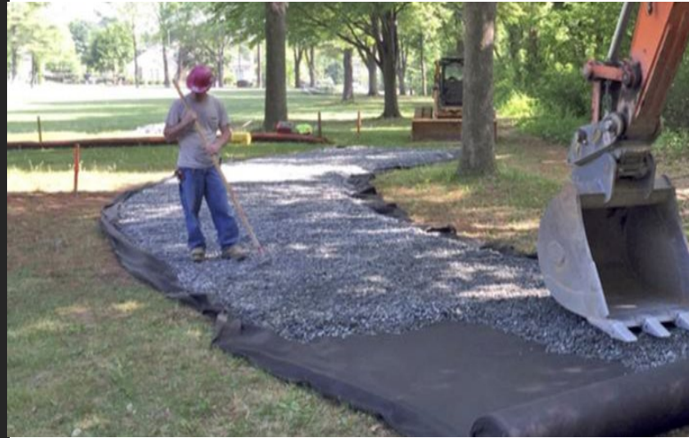
PLACE GEOTECH FABRIC AND STONE BASE
