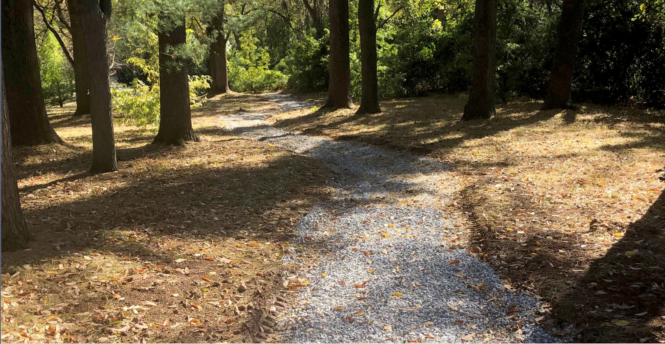
Hoops Park – West Chester, PA 4,400 sq. ft. trail Managing stormwater with an inclined perkE-pave trail
