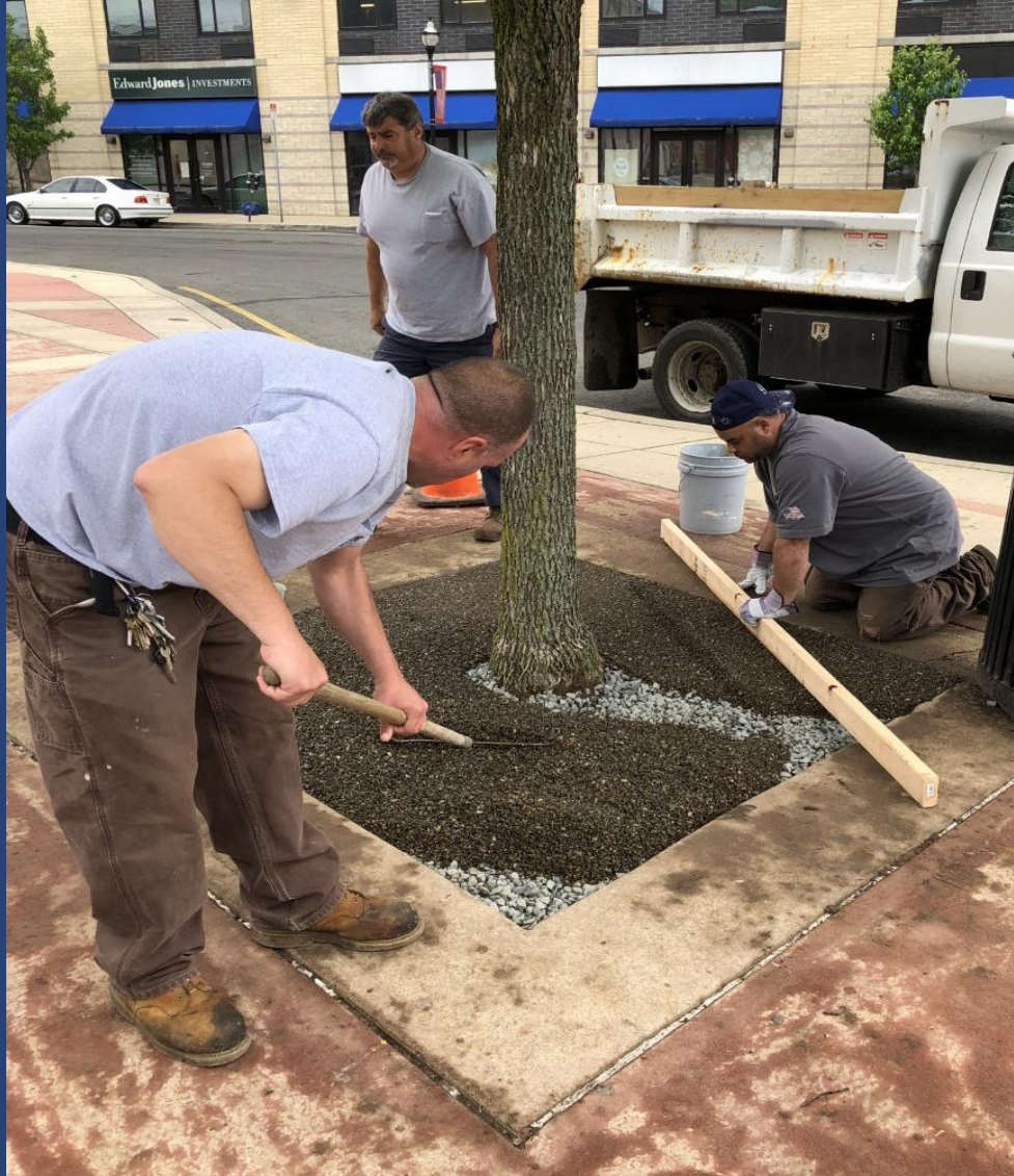
Pour, rake and screed material.
