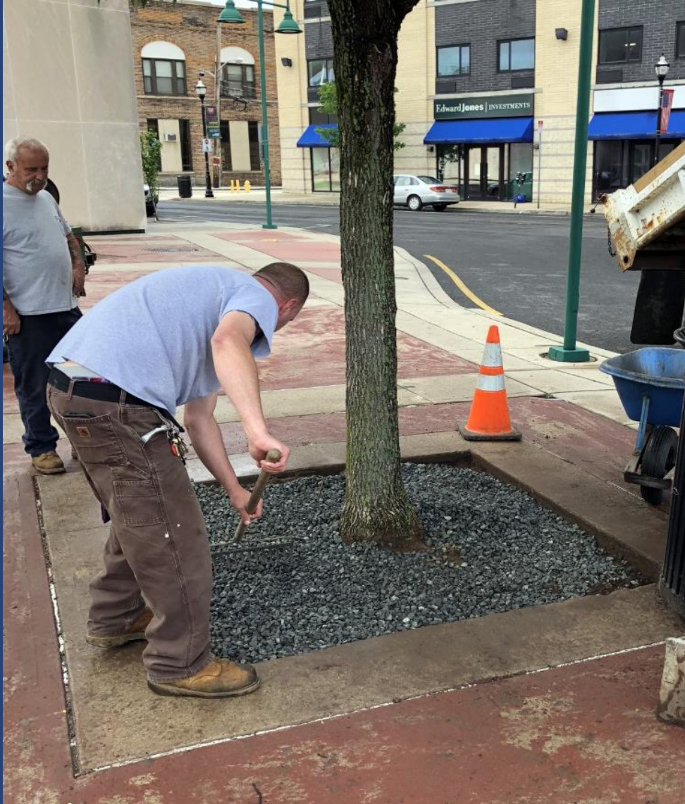
Place and tamp CLEAN 3/8-1/2 stone to an elevation of 1.5" below finish
