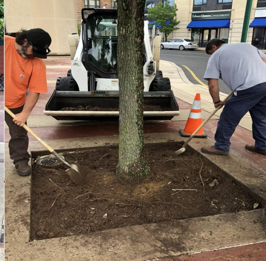
Remove soil to a maximum depth of 4" where possible; without damaging tree roots
