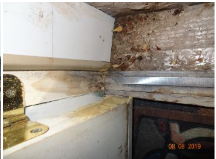
water stains and rot at rear basement door frame and door
