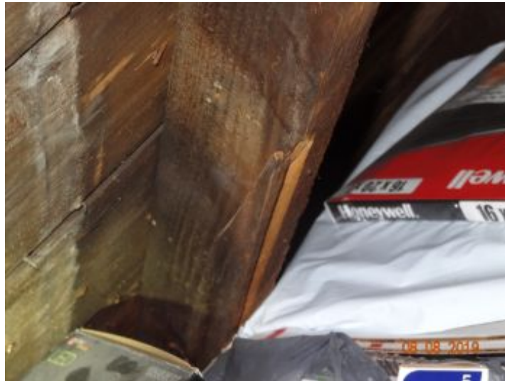
damaged rafter
