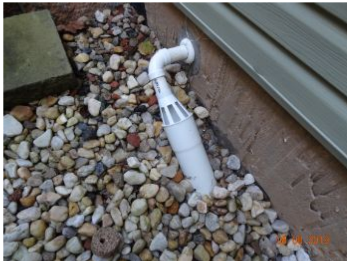
unknown pipe penetrating foundation wall/possible sump pump
