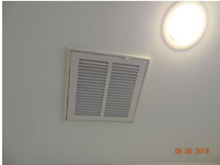
central a/c returns/air filters
