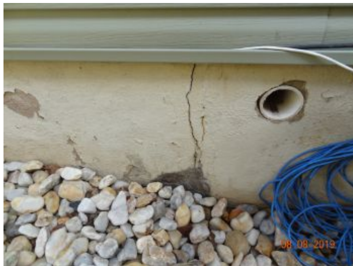
crack at right side foundation wall.
