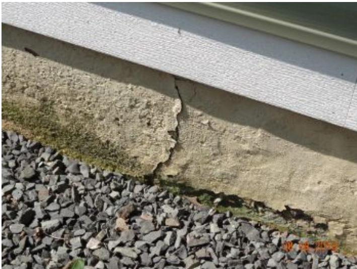
crack at left side foundation wall.
