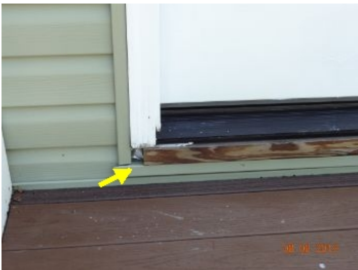
small openings at base of front entry doorway
