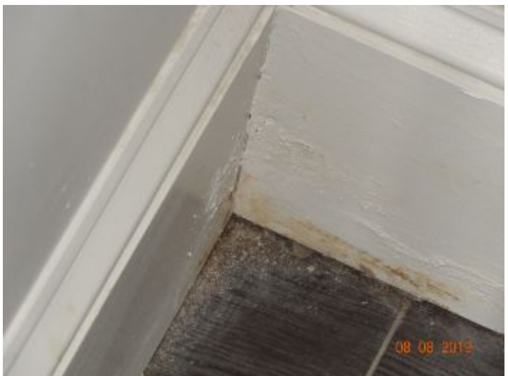
Water stain at base trim behind washing machine
