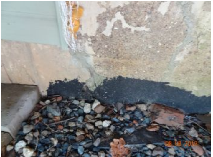
opening at base of foundation wall between new and old foundation walls/low spot at grade
