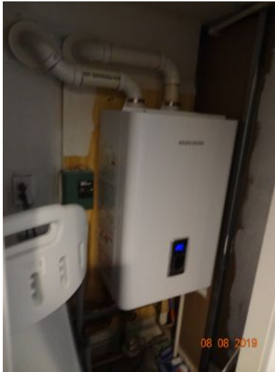
tankless boiler/water heater
