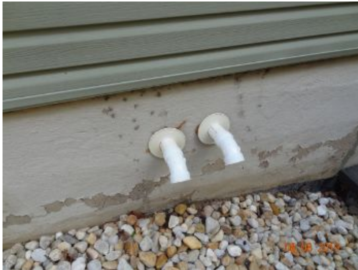
tankless boiler direct vents
