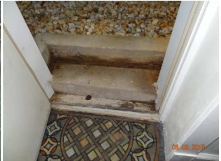
no floor drain at exterior of rear basement door
