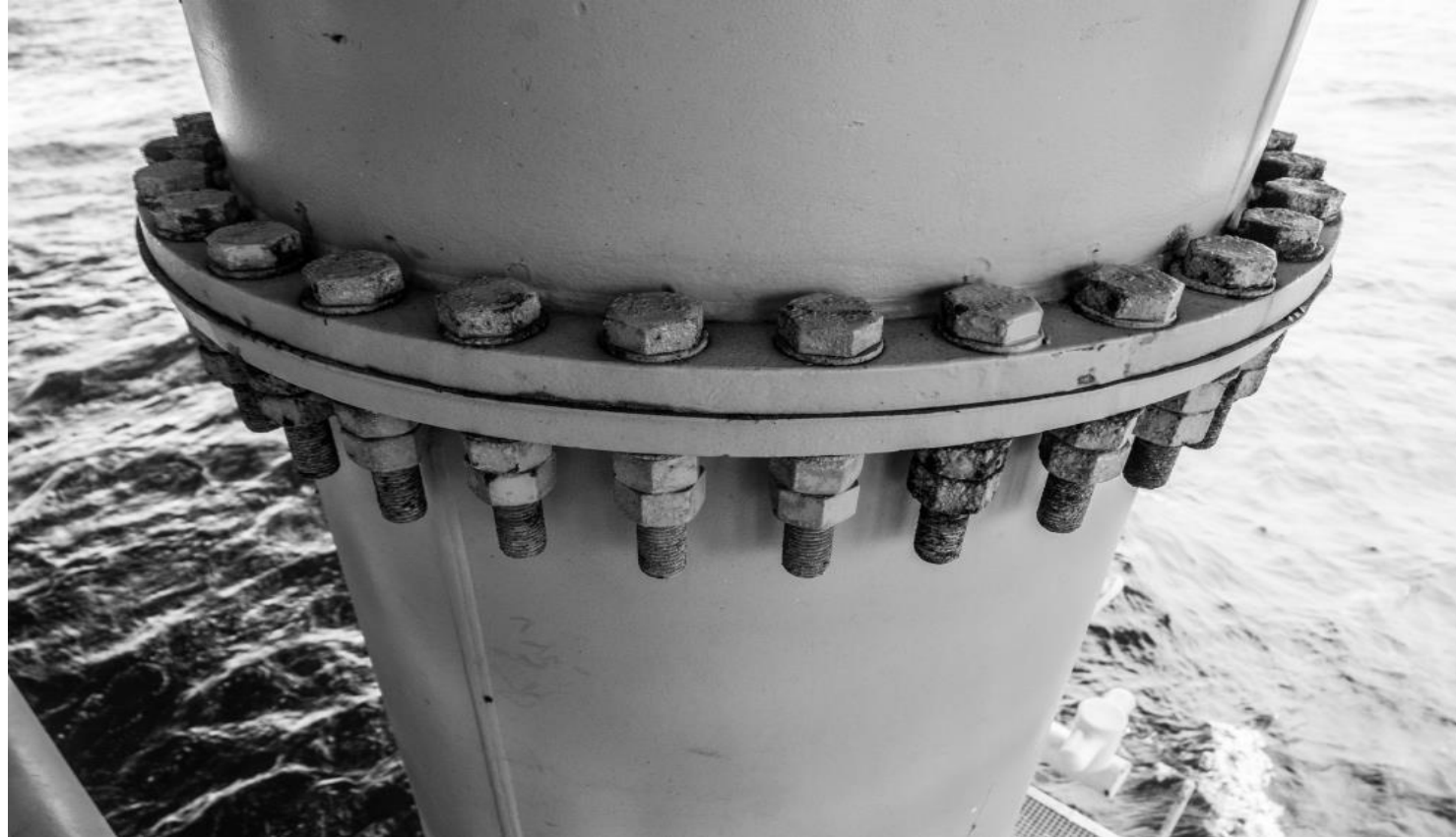
BOLTING – TEMPORARY METHOD
