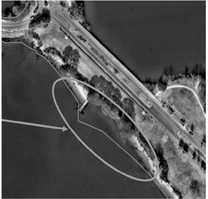
20 years of erosion can be seen at the foot of Lions Bridge Dam.
