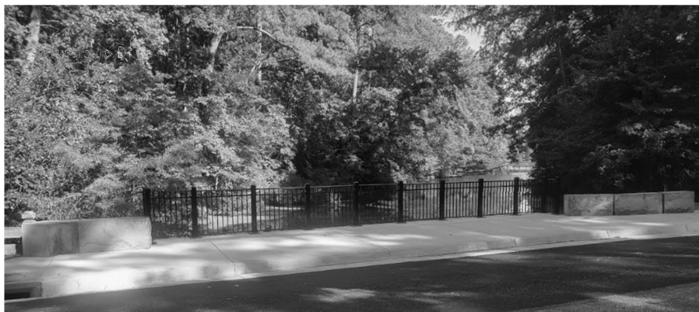
The sidewalk drain roadwork in front of the Mariners' Museum is complete.
