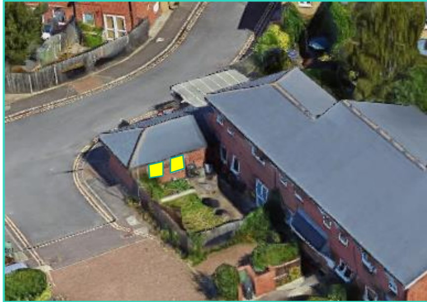
Image 7.8 – Photograph showing the two overhung ground floor windows (highlighted in yellow)
