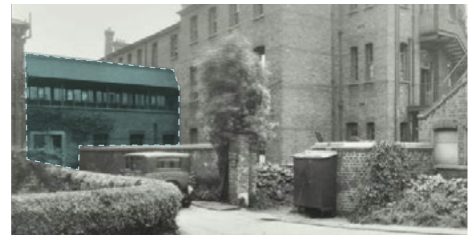
Link Building Connected to Block 'C'
