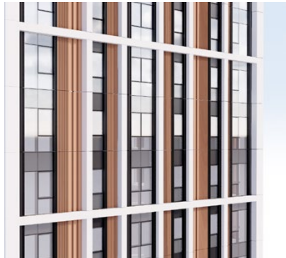
View of north western facade
