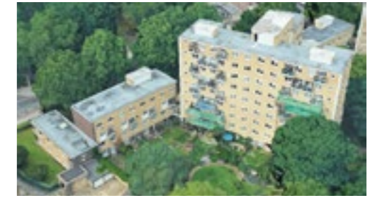
2. Post War Slab Blocks
