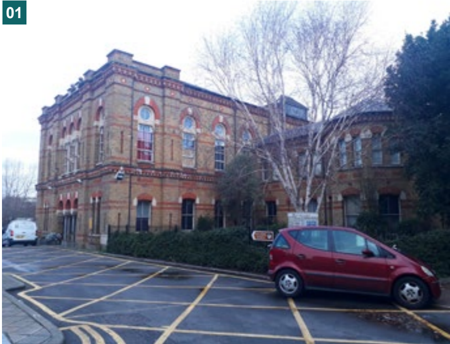
View of the Masters House from Site Entrance
