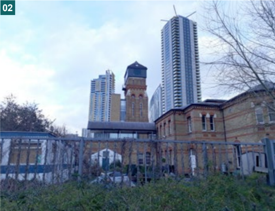
View of the Water Tower
