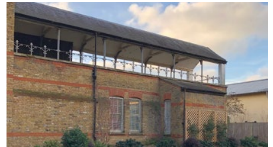
Rear View of Remaining Link Building
