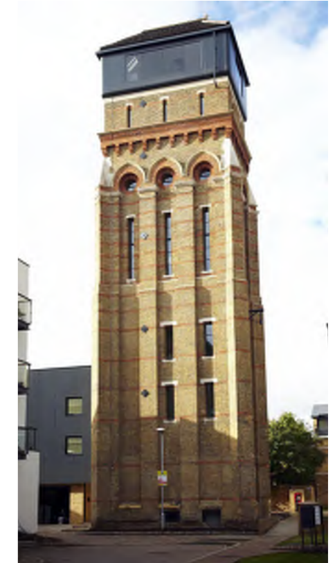
Grade II listed Water Tower
