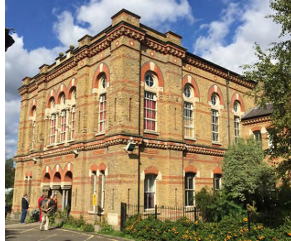
Grade II listed Administration block to former Workhouse
