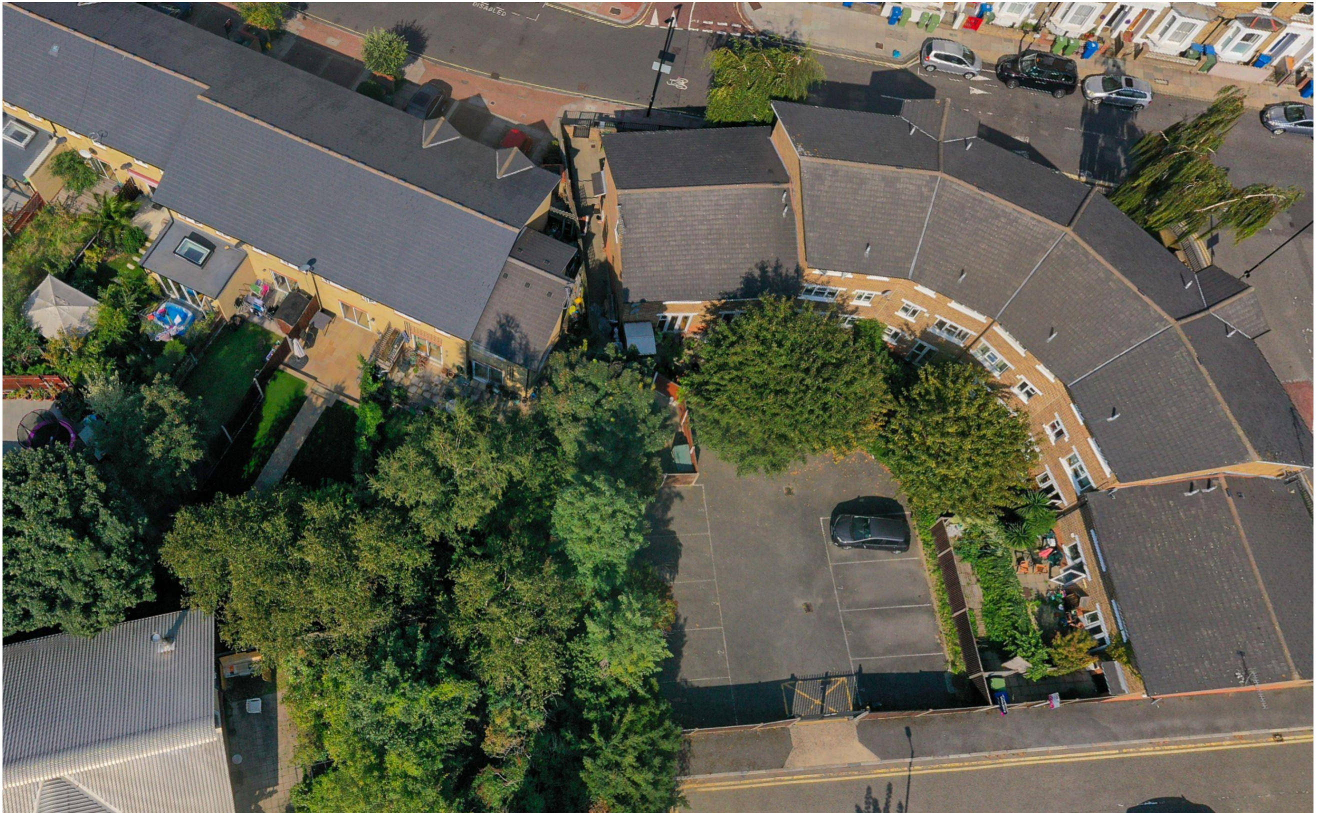
Aerial Drone Photograph 4 - 16.09.20
