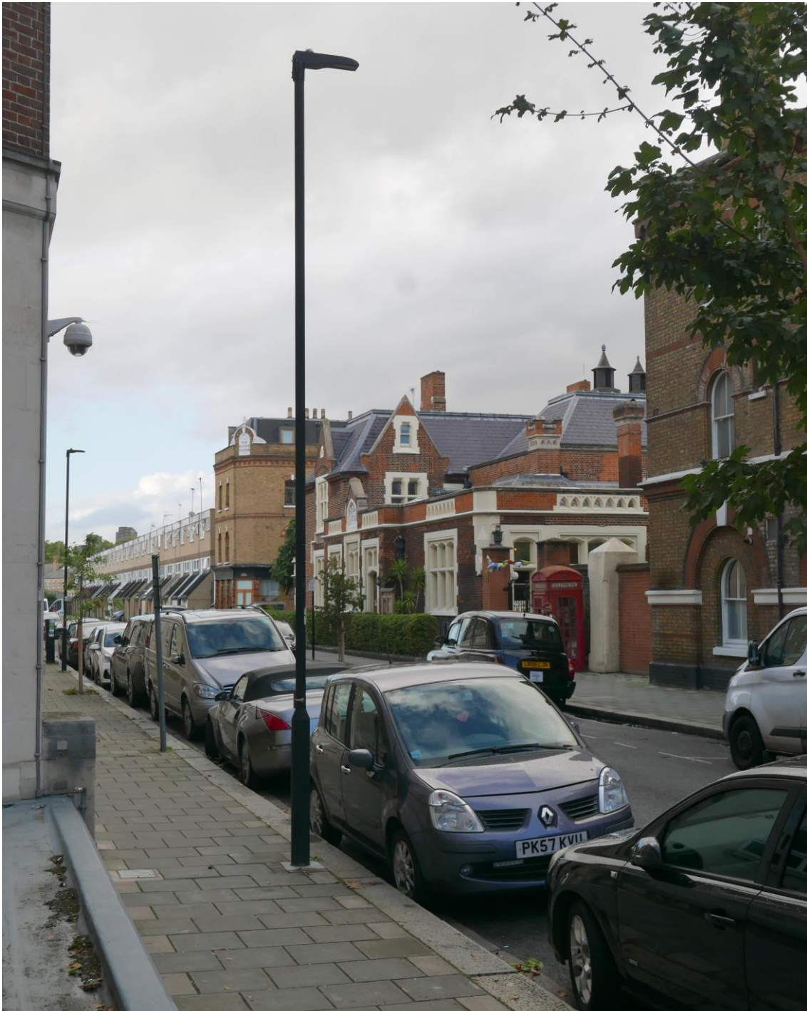
The locally former Court Tavern Public House, the listed former Magistrate's Courthouse and the listed former Fire Station in Renfrew Road. View from the south, showing their unbroken roof-lines.
