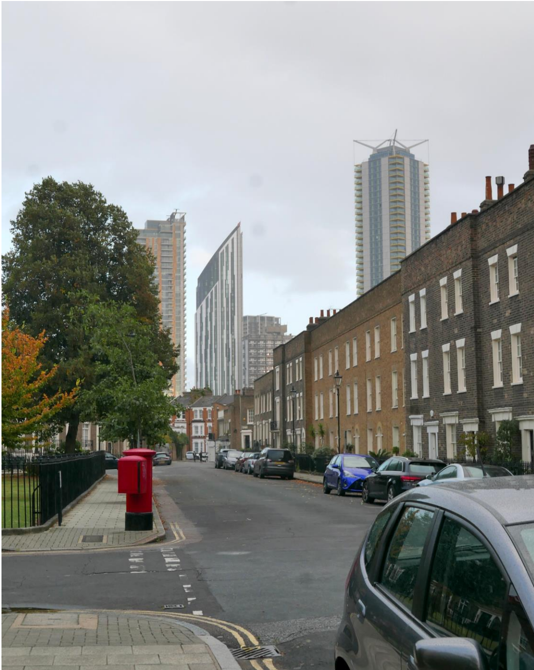
View eastwards along the south side of Walcot Square showing the highly damaging impact of poorly considered tall-building development on the settings and significance of listed and other buildings within the conservation area and on views out of the conservation area.
