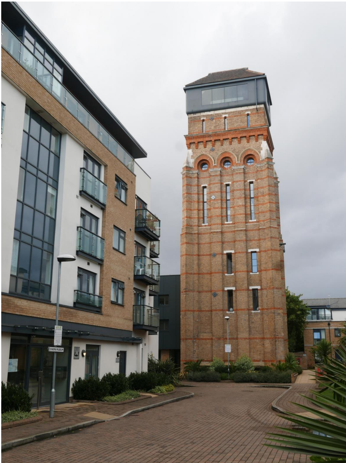
The listed former Water Tower of the former Lambeth Workhouse and Hospital. View from south-east showing its present distinctive and uninterrupted profile.
