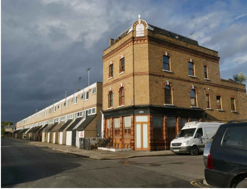
The locally listed former Court Tavern Public House at the corner of Renfrew Road and Dugard Way and the three-storey housing along the north-east side of Renfrew Road. View from the south showing their present uninterrupted roof-lines.
