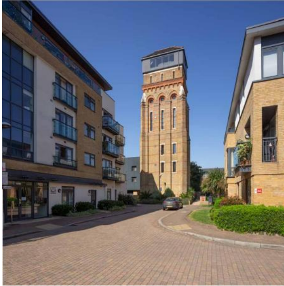
Figures 12a to c - Existing views showing the kinetic experience as one moves west along George Mathers Road
