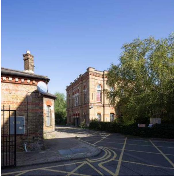
Figures 10a to 10c - Existing views of Master's House showing the kinetic experience of approaching the building
