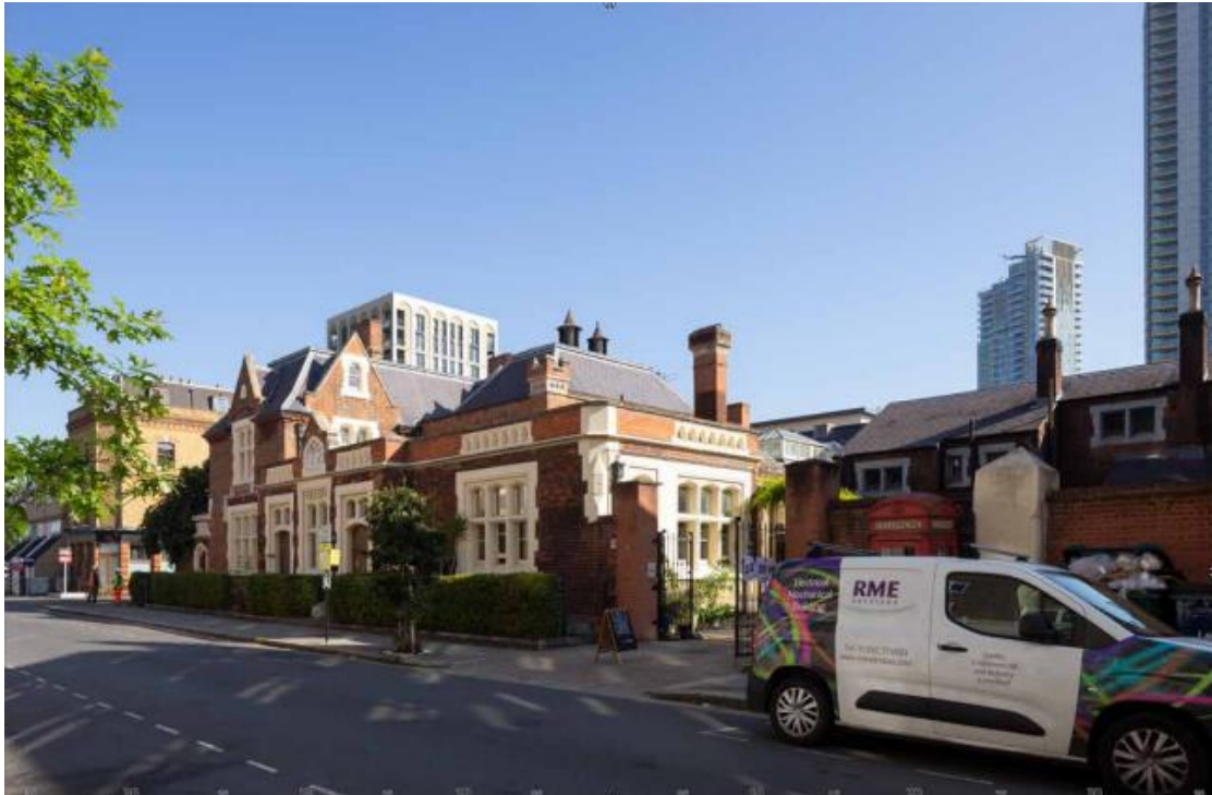
Figure 15 – Proposed view of the Former Lambeth Magistrates Court. The former Court Tavern public house is visible on the far left
