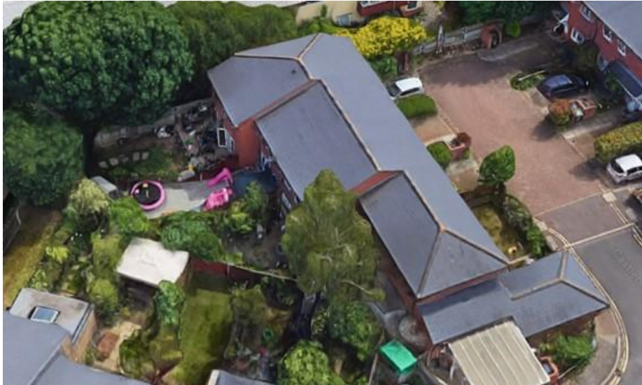
Figure 42 – Properties on Castlebrook Close. 1 Castlebrook Close is at the bottom. 4 Castlebrook Close is at the top
