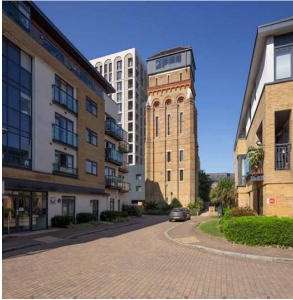
Figure 13a to 13c - Existing views showing the kinetic experience as one moves west along George Mathers Road
