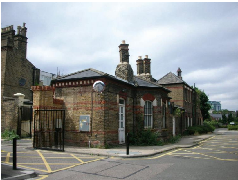
42 Renfrew Road (former Court Tavern Public House).
