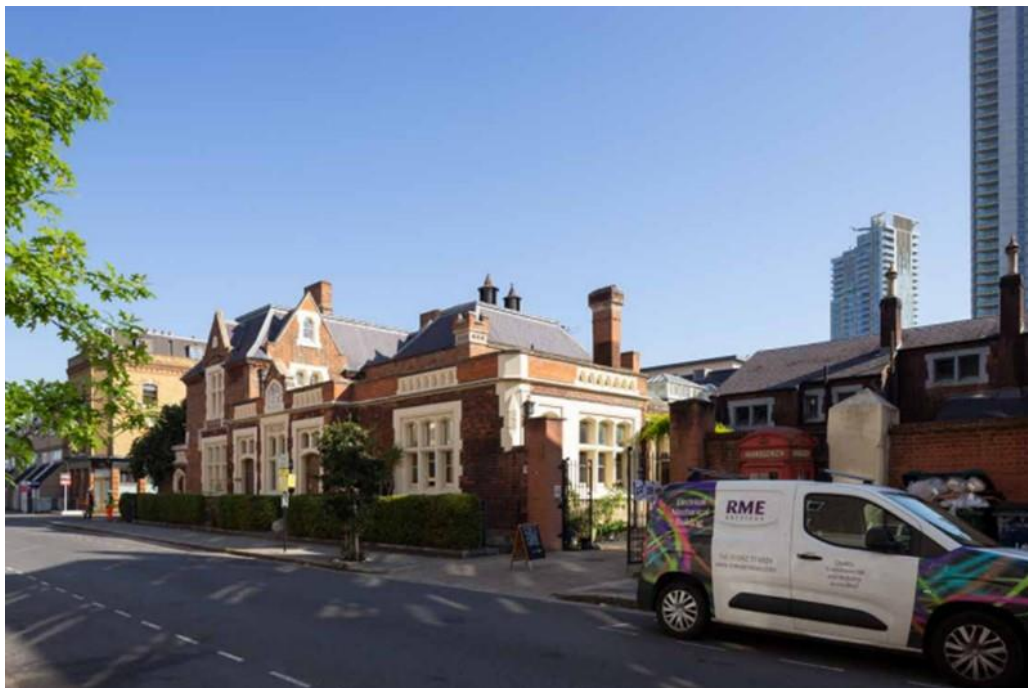
Figure 14 - Existing view of the Former Lambeth Magistrates Court
