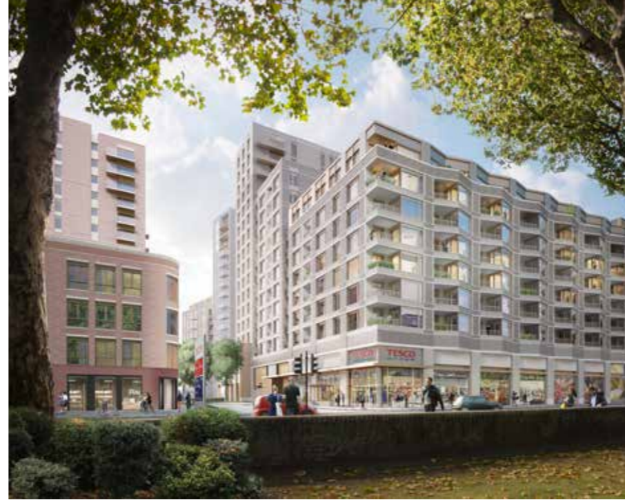
Tesco Kennington Lane (on site)
