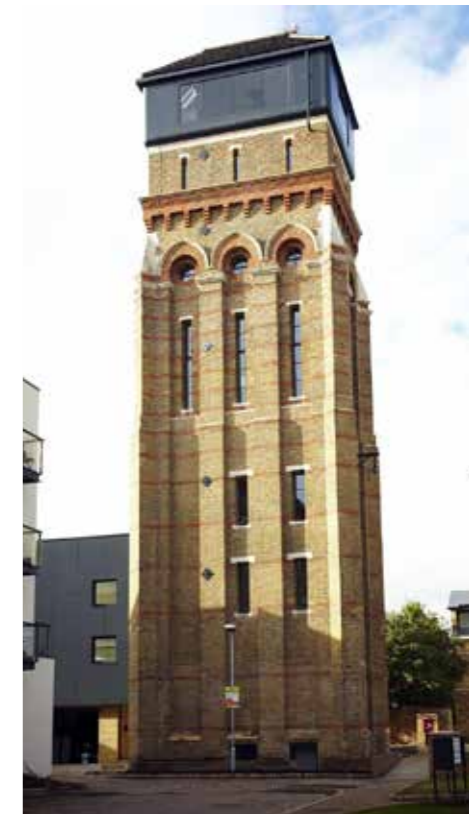
Grade II listed Water Tower
