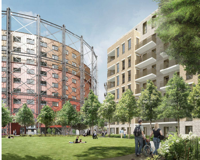
Oval Gas Works (on site)
