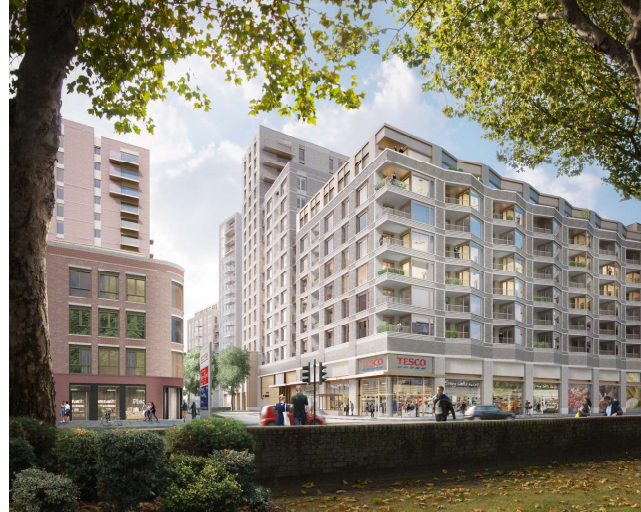
Tesco Kennington Lane (on site)
