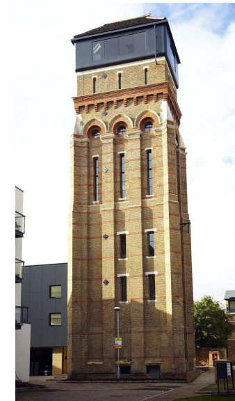
Grade II listed Water Tower
