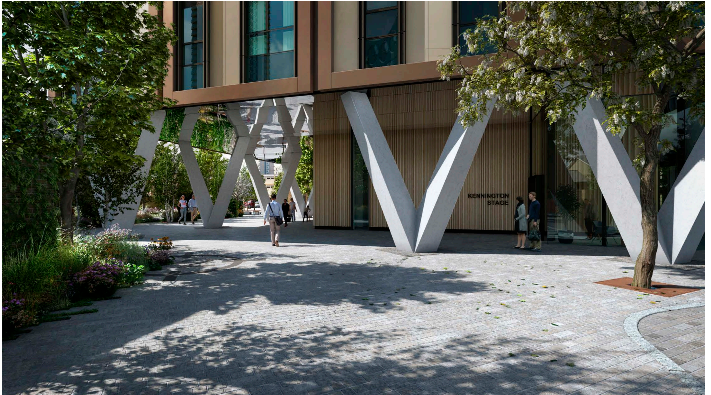
Figure 18 - View looking underneath the covered walkway along the public route arriving from Longville Road leading towards Dugard Way
