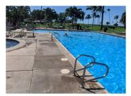
Pool tile was installed in 1997 and has a useful life of approximately 20yrs, however the life can be extended with repairs. Repairs to be performed this summer when pool is drained.
