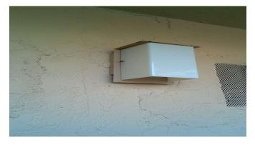
The hallway lighting is original and reaching the end of its useful life. Recommend replacement with energy efficient lighting. It is not overly inefficient and is more a cosmetic repair.
