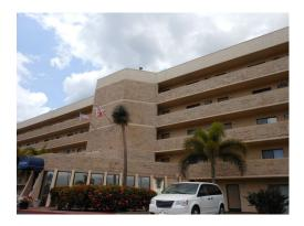
The full exterior of the building should be painted to protect against concrete spalling. The brick and morter exterior is not a waterproof surface and concrete spalling has begun to take place. To preserve the building and protect against spalling the full exterior should be painted. The building ends that face the ocean should be waterproofed every 5 yrs. Much of this work can be performed by in house painting. Per Board, this was completed in 2014 for approximately \$60,000.
