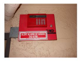
Per the previous reserve study the fire alarm pull stations, bells and flashers were replaced in 2003. Future replacement cost will increase as codes have changed require replacements to include alarm bells in each unit.
