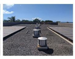
The roofing system was installed in 1989. The membrane was covered with gravel to protect the surface from the UV rays that cause roofing materials to break down. This surface should last 40yrs or longer.
