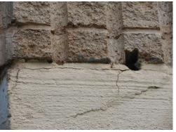
Concrete spalling occurs when moisture and oxygen penetrate through the pores of concrete to
