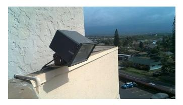
The parking lots are lit by 7, 400 watt HPS flood lights. These lights are reaching the end of their useful life and should be replaced with more energy effeciant lighting.
