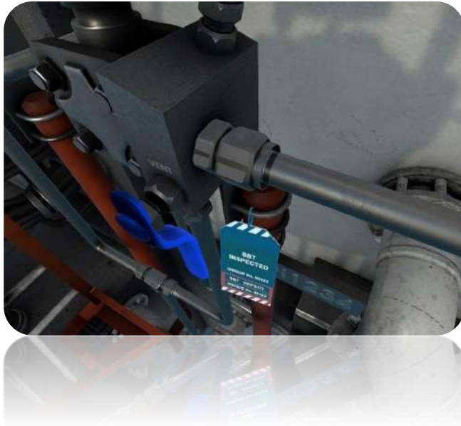
Figure 6 - The inspection tag should be fitted before the pipe is disassembled.
