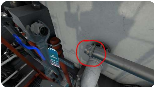
Figure 14- The Ferrule and source of the fault. The trainee should inform the System Manager that the fault is: "There is debris on the front ferrule" via the radio.
