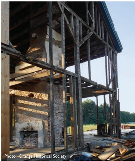
The original bricks (right) from the chimney/fireplace (left) of the Alling Inn will be reused on the new chimney and will also cover the foundation in the back of the house.
