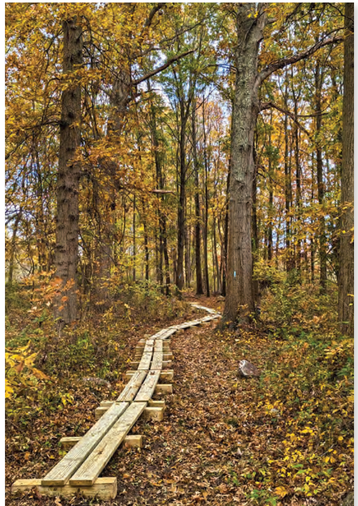
Bogwalk that was constructed for the Paugussett Trail at the Wiacek Meadows Open Space.
