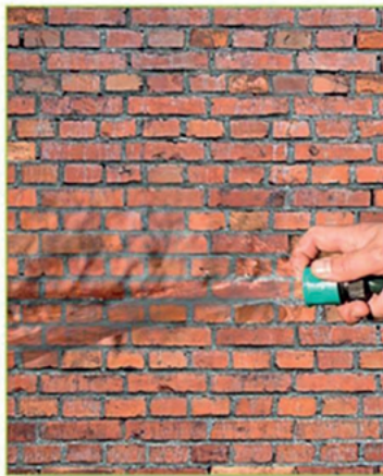
Step 02 Wetting Wall Surface
