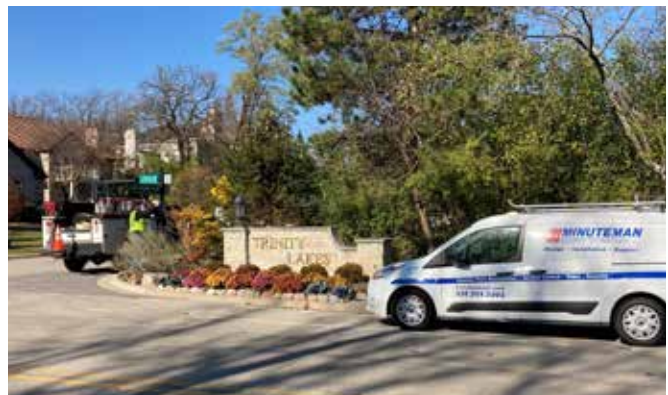
LPR Cameras Being Installed at Trinity Lakes Subdivision
