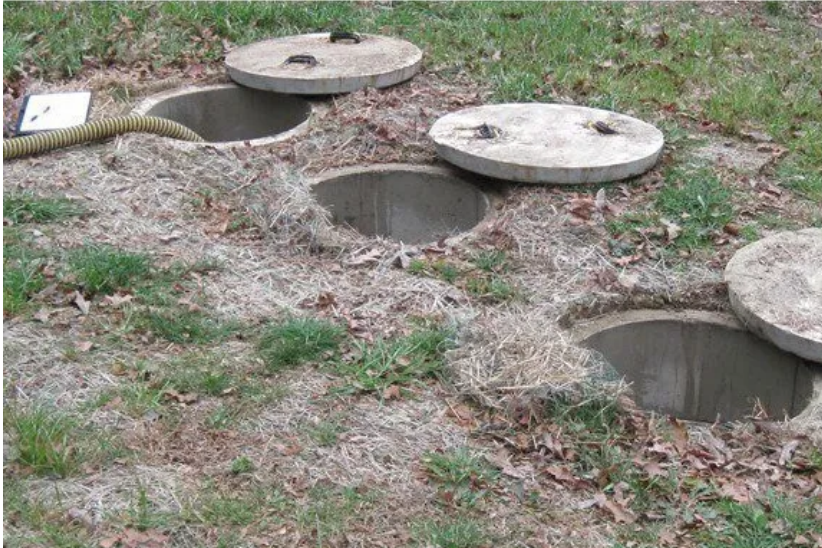
Newly installed three chamber septic and pump tank (Photo by Amy Galford)
