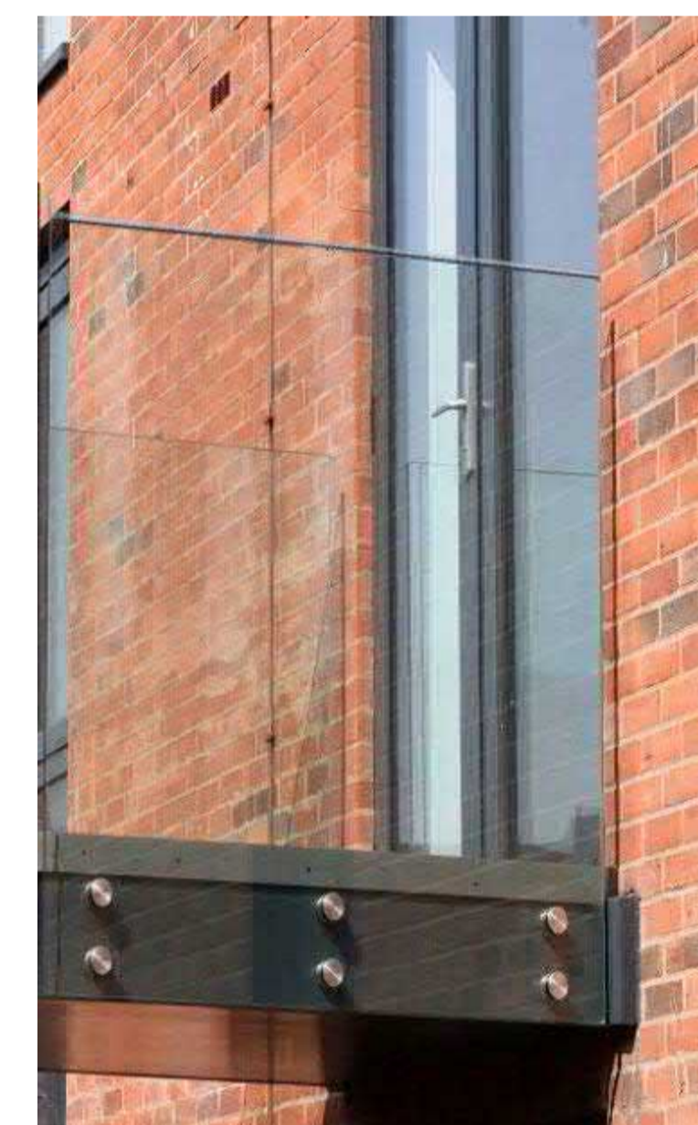
Laminated glass balustrade with PPC handrail, colour RAL 7015
