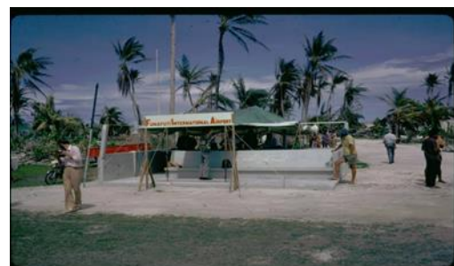
Funafuti airport after Hurricane Bebe 1972
