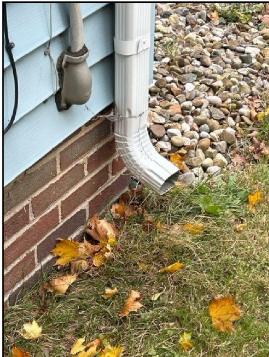
9. Downspout is not directed into its proper...
