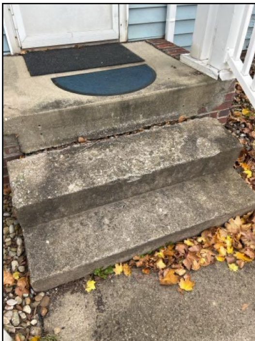
24. Steps or landings settling or heaving
