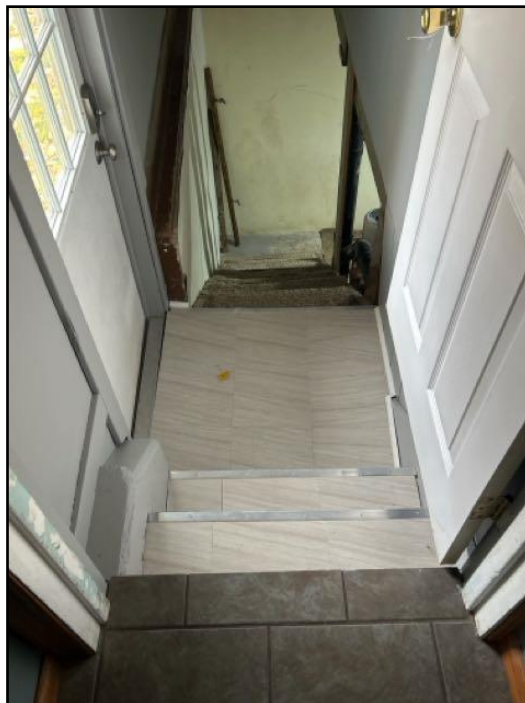
86. Recommend installing handrails for safety.
