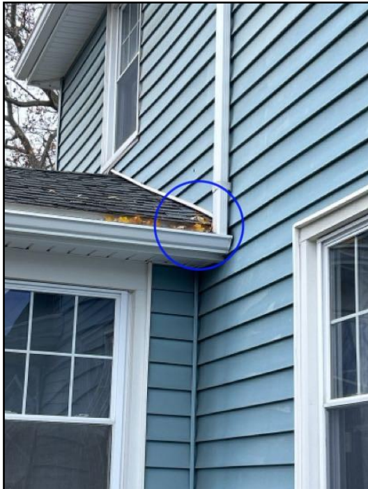
4. Monitor for overflowing water and install...
