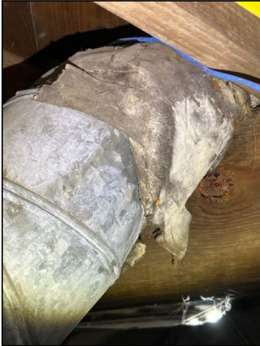
56. The white tape covering some of the joints...
