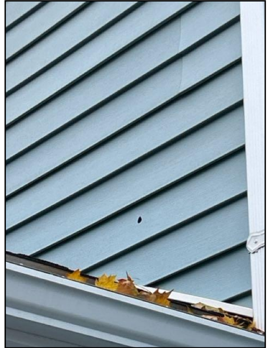
13. Typical mechanical damage noted in areas....
