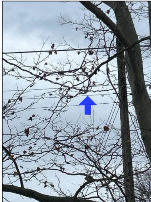
50. The service wire is in contact with tree...
