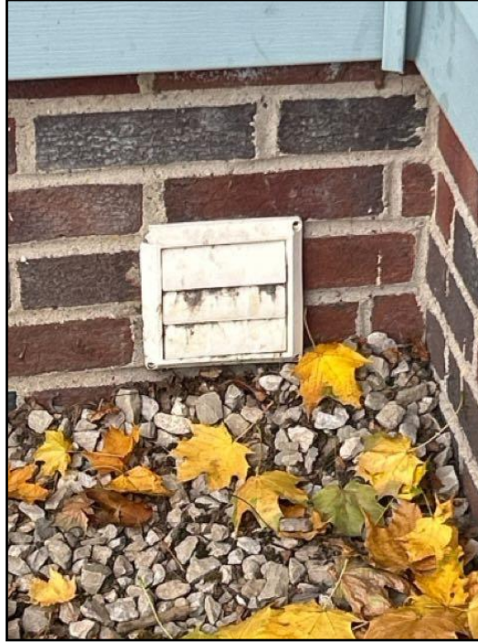
3. Vent close to grade. This could easily be...
