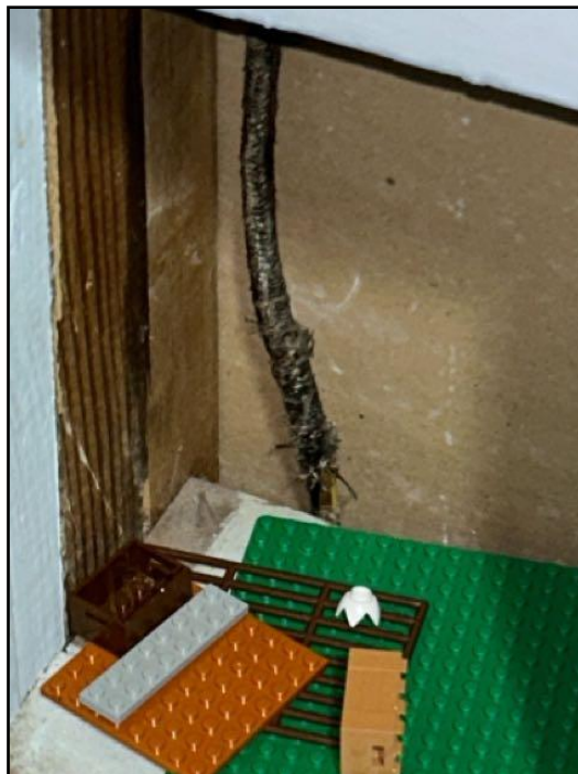
53. Spliced/damaged wires. Replace or install...
