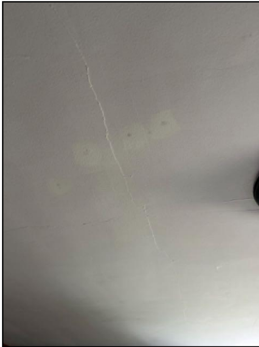
70. Cracked areas. Prior repairs noted. Monitor...
