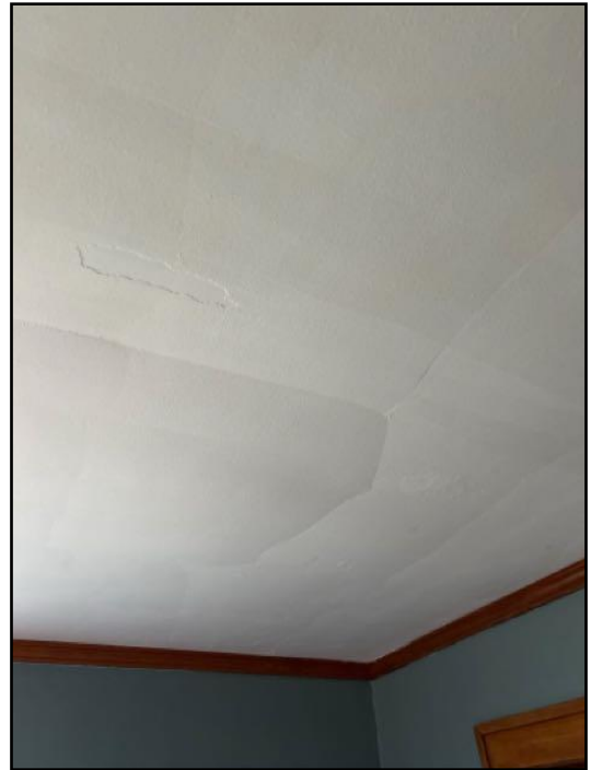
71. Cracked areas. Prior repairs noted. Monitor...
