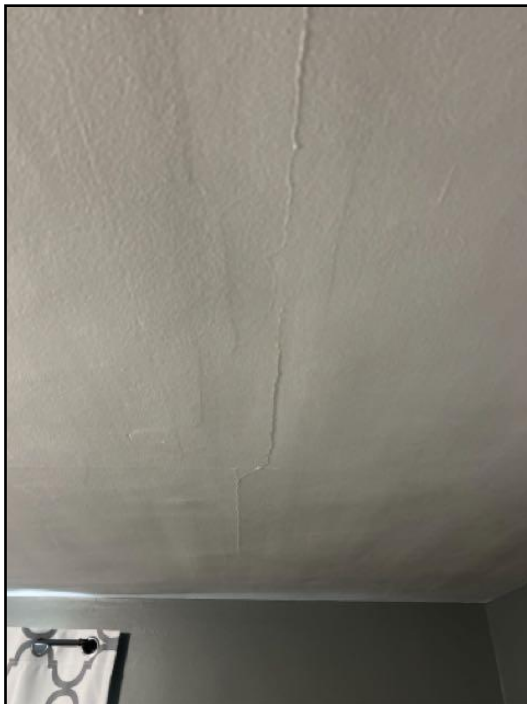
68. Cracked areas. Prior repairs noted. Monitor...
