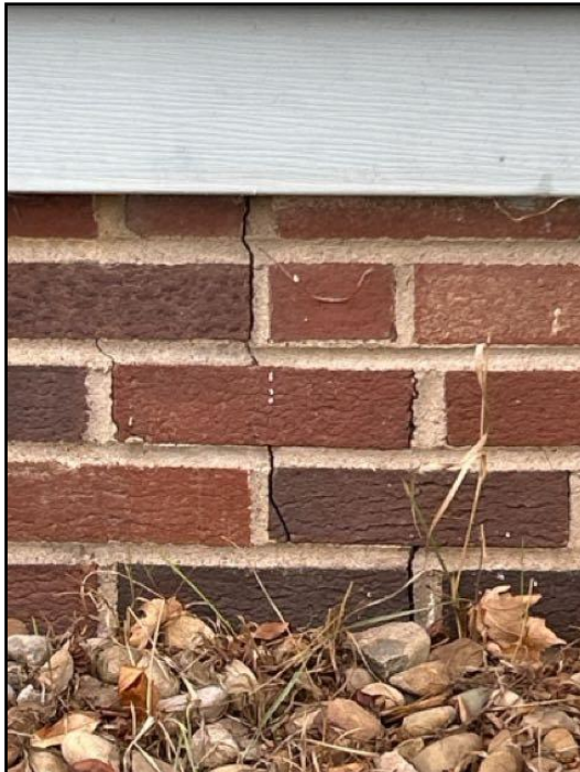
43. Crack(s) noted on the basement foundation....
