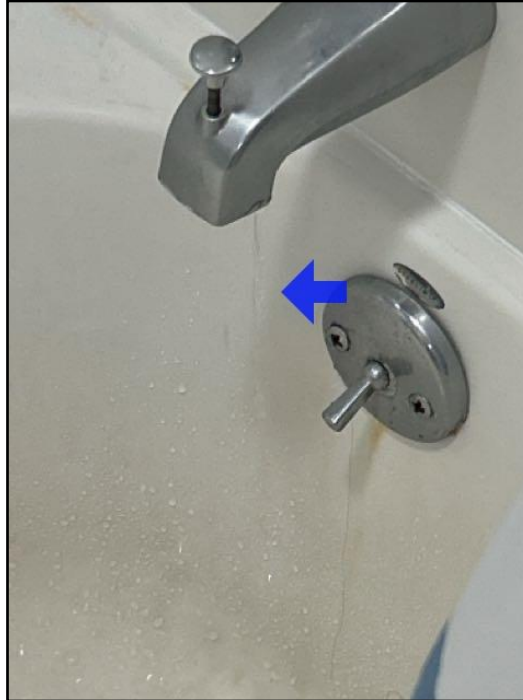
66. The shower diverter leaks while the shower...
