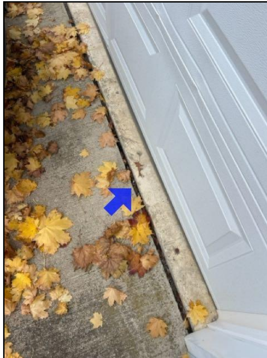
27. Recommend sealing the expansion joint at th...
