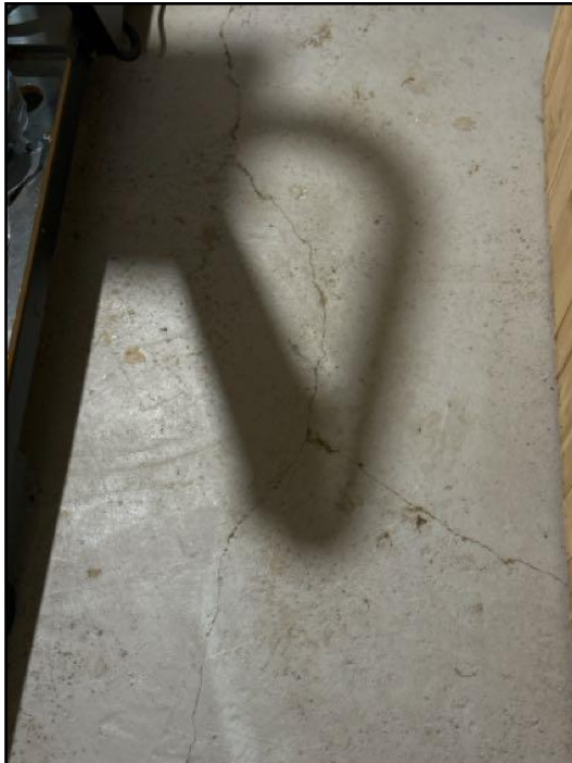
80. The basement floor is cracked in areas....
