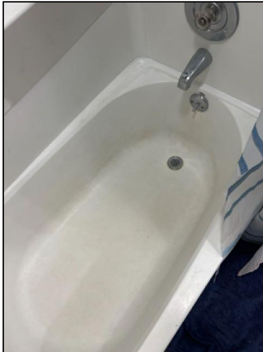
67. Surface defects. Clean or replace as needed.
