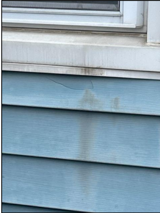
12. Typical mechanical damage noted in areas....
