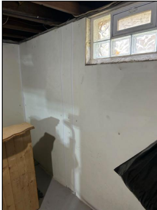
88. Prior B-Dry type repair noted along the...
