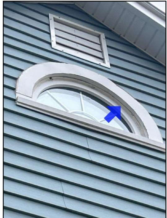
18. Paint and caulking needed on window(s).
