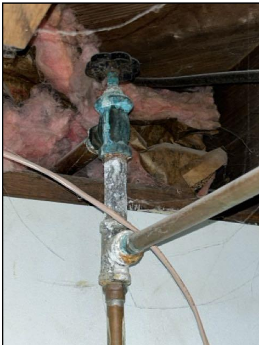
61. Corrosion/Calcium buildup noted on some...
