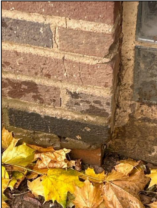
41. Crack(s) noted on the basement foundation....
