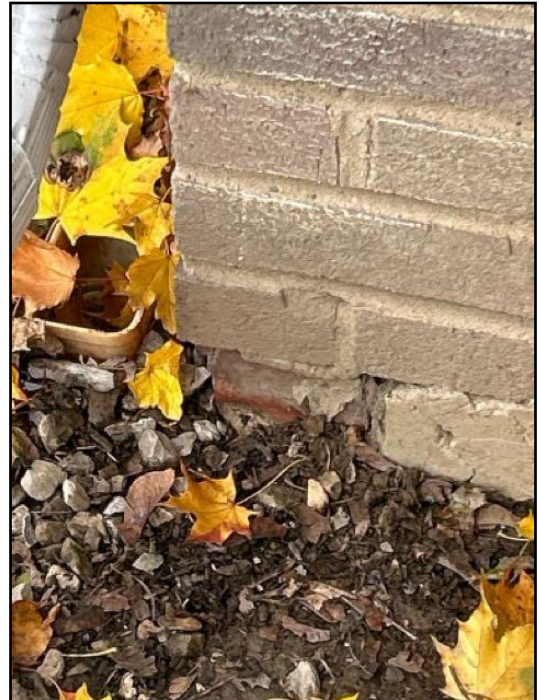
42. Crack(s) noted on the basement foundation....
