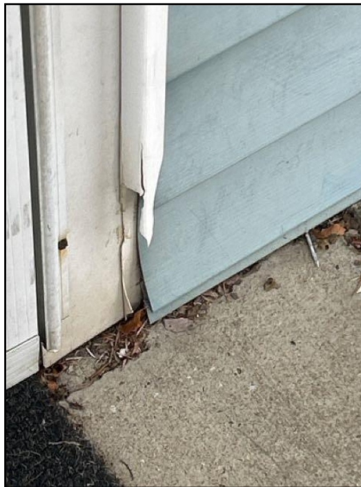
14. Typical mechanical damage noted in areas....
