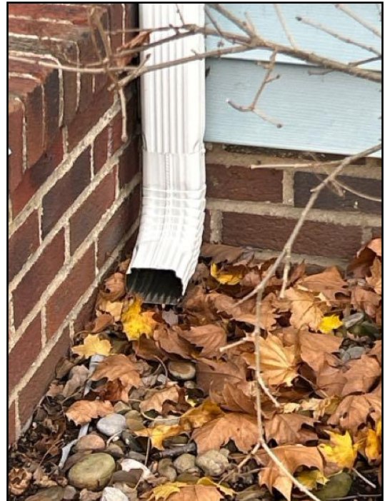
10. Downspout is not directed into its proper...
