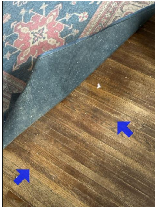
78. Ghosting noted on the floor. Repair area as...
