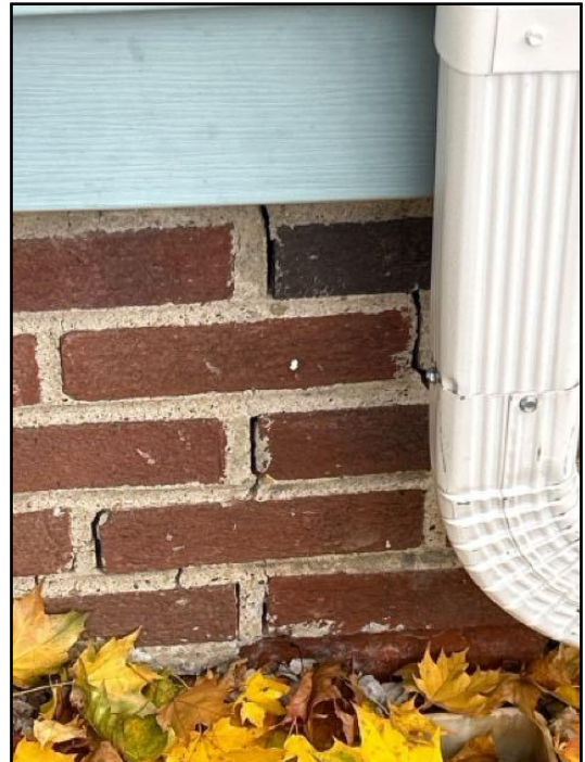
40. Crack(s) noted on the basement foundation....
