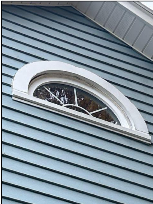
17. Paint and caulking needed on window(s).
