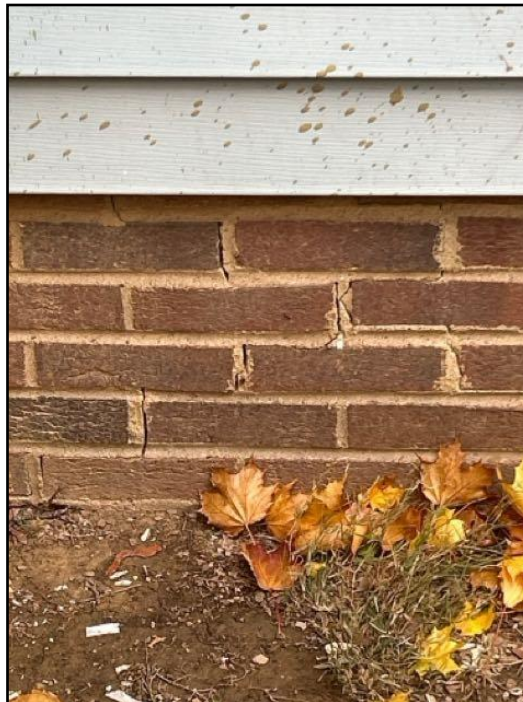
45. Crack(s) noted on the basement foundation....
