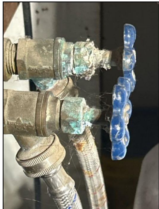
62. Corrosion/Calcium buildup noted on some...
