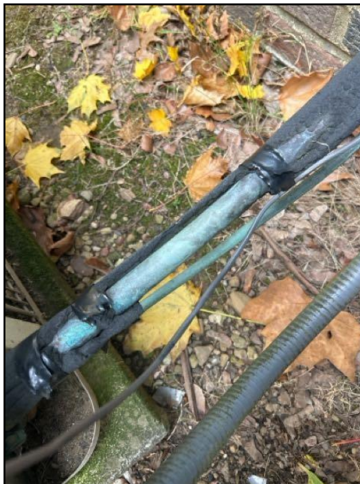
59. Damaged Insulation on the refrigerant line....
