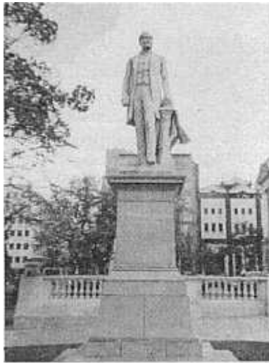
Sir Edward James Harland Engineer and Shipbuilder And M.P. for Belfast-North 1895
