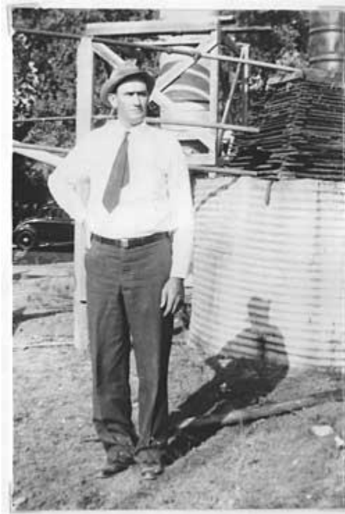
Thomas Daniel Harlan stands beside the cooling tower and cistern outside of his cotton gin sometime during the 1930s. Water was used to cool the diesel engine that powered the gin's machinery. The gin crew took baths in the cistern because the water was warm and fairly clean.
