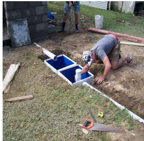
BIPU installation Fiji
