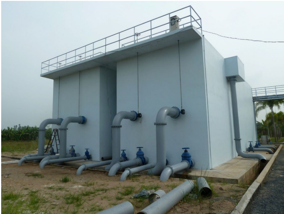
Compact design includes filter with in-filter backwashing, no pumps required
