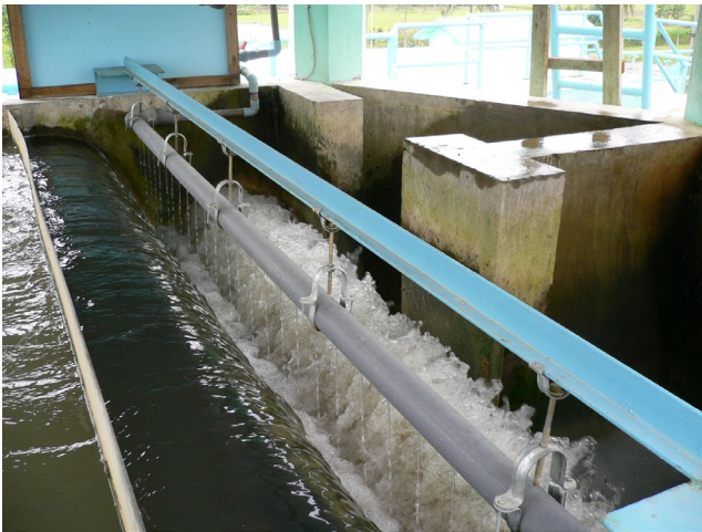
Efficient Mixing weir, 1 second only
