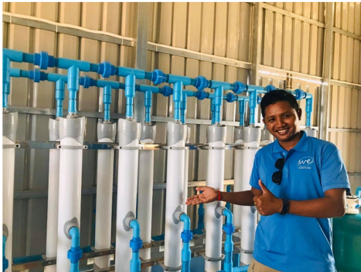
Newly developed sUF-MMU-SDE with capacity of 12 m 3 /h in Cambodia
