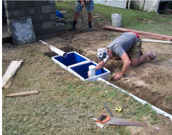
BIPU Lego style wastewater treatment
