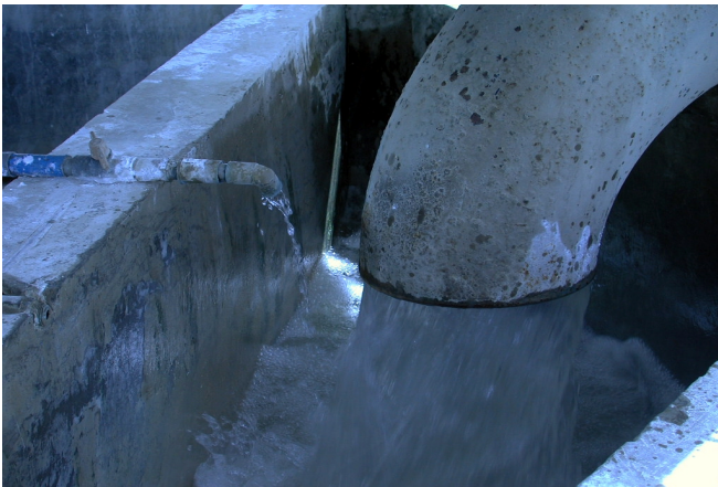
Poor mixing before revamp
