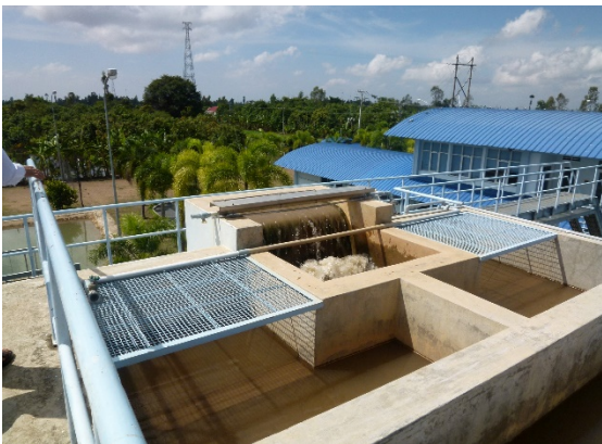
Mixing and flocculation stage 30% of space
