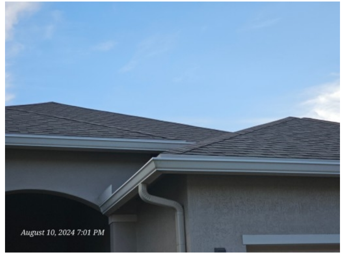
Roof Coverings - Asphalt shingles, Dimensional/architectural
