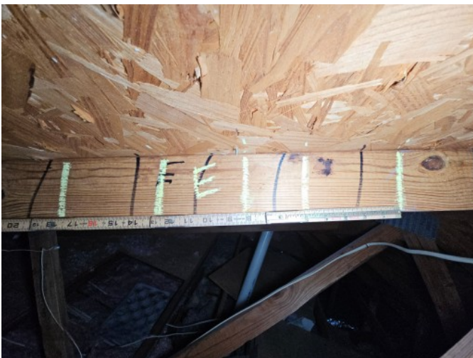
Roof Deck Attachment - 6" spacing on the edge
