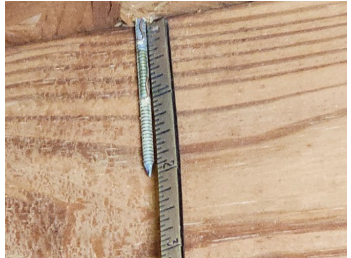
Roof Deck Attachment - 8d ringshank nails
