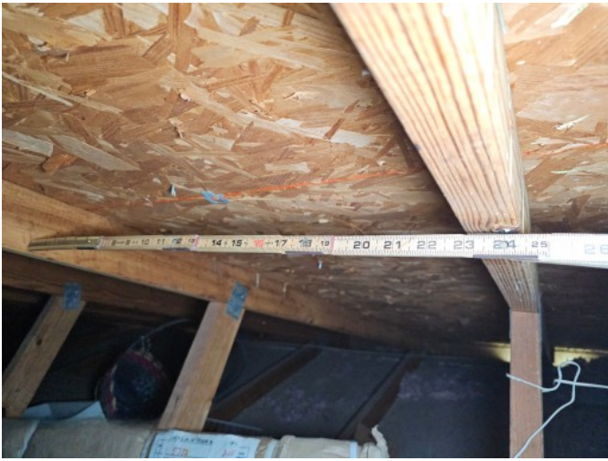
Roof Truss Spacing - 24"
