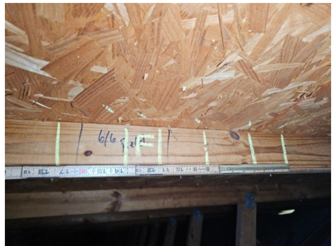
Roof Deck Attachment - 6" spacing on the field
