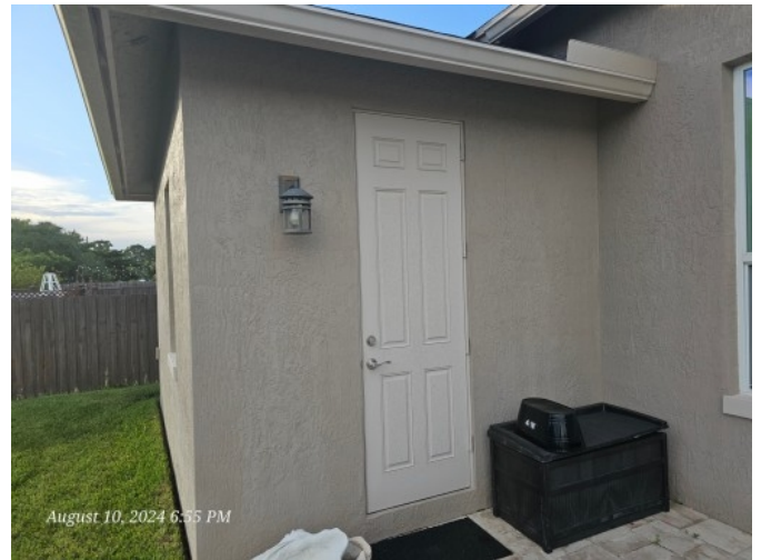
Back Elevation - entry door is impact rated
