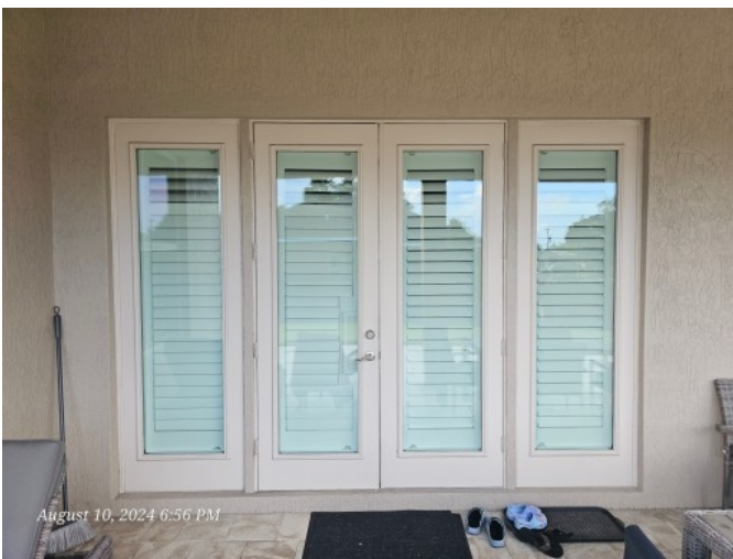
Back Elevation - windows are impact rated, glazed entry door is impact rated
