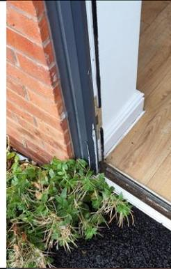
Weep holes are missing from underneath the living room window.
