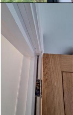
A close-up photograph of the top edge of a door frame. It shows a wooden door with a metal hinge. On the right side, there is a fire and smoke seal. On the left side, there is a fire seal. The seals are not consistent in appearance and are nailed into the frame. |  |
