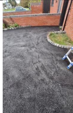
There are no edgings on the left-hand side of the door to hold the tarmac in place.
