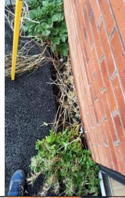
There are no edgings on the left-hand side of the front room window to hold the tarmac in place.
