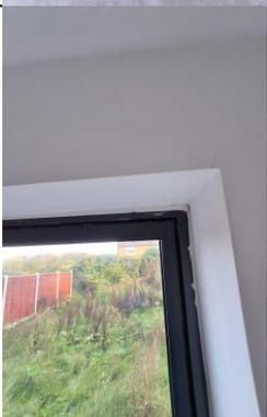
A close-up photograph of the top edge of a bi-fold door frame. A thick, uneven layer of mastic sealant is visible, which is significantly larger than the standard gap, indicating a poor installation.                                                                 |  |
