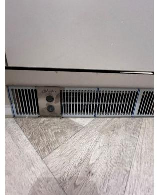
Plinth needs securing properly with clips and there is rubbish behind that needs cleaning out
