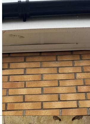
The window sill cover end caps are all loose and need to be glued/fixed into position
