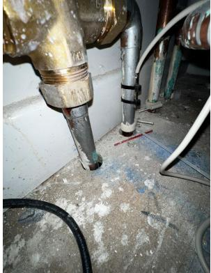
Fire stopping to floor penetrations required here
