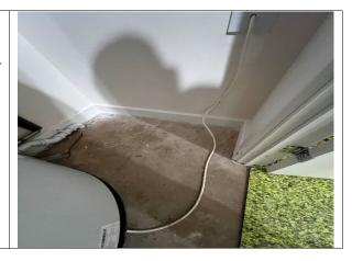
This waste pipe that penetrates the floor will need to be properly fire stopped as well as the other penetrations in the photo bottom photo.
