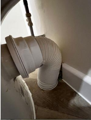
Plastic needs to be removed from behind the waste pipe and properly filled and decorated
