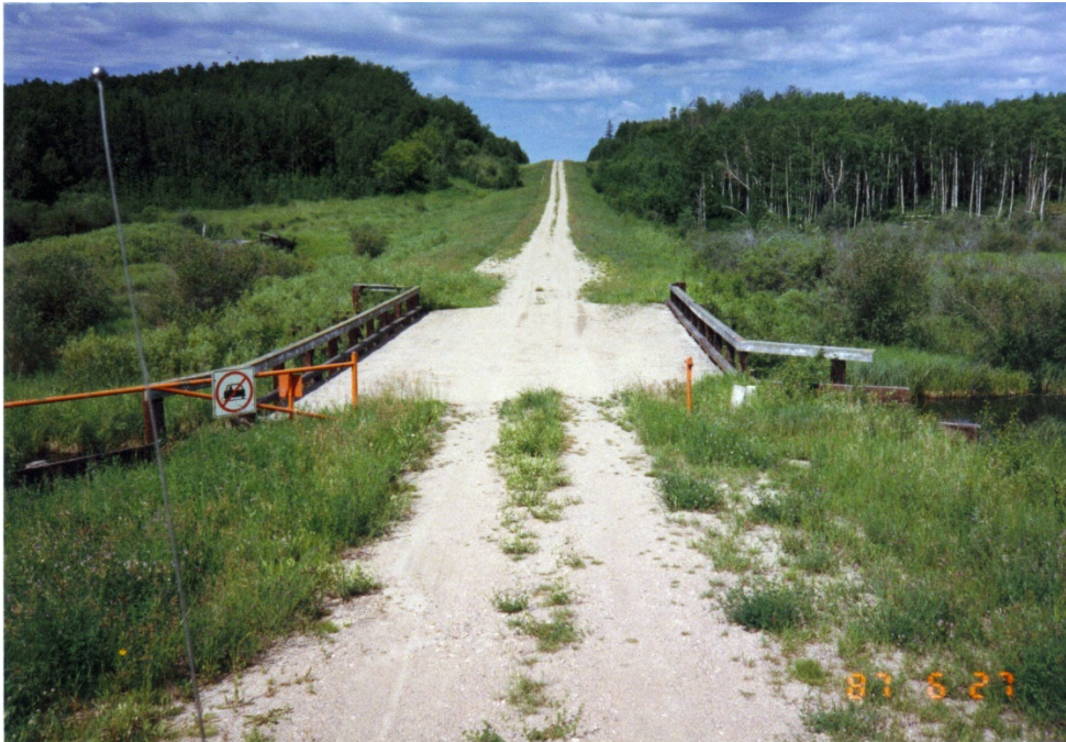
Bridge over Sturgeon River West side prior to road closure
