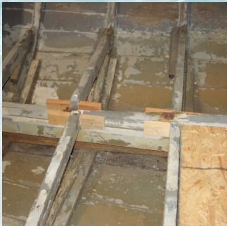
Frames required added support; floorboards required repairs and priming.
