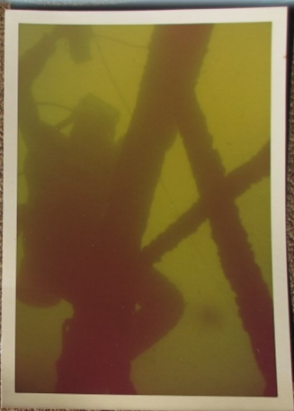
Three span bridge under 50 feet of water just west of the Conklingville Dam. The dam was built as a work project during the 1930's. This site is west of Albany.
