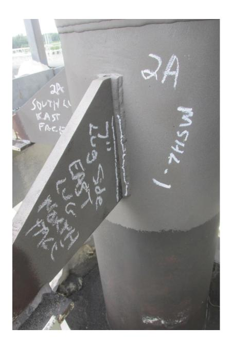
**Figure 1.** Shown is the north side of the east support lug **and a set of the indication detected during a non-destructive inspection outlined in white.**
