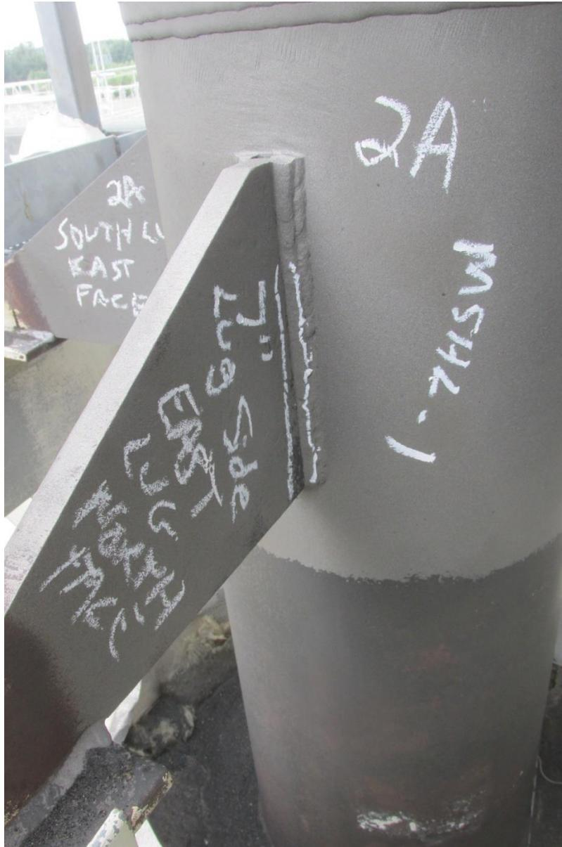
**Figure 1.** Shown is the north side of the east support lug [REDACTED], with the approximate location of the indication detected during a non-destructive inspection outlined in white.
