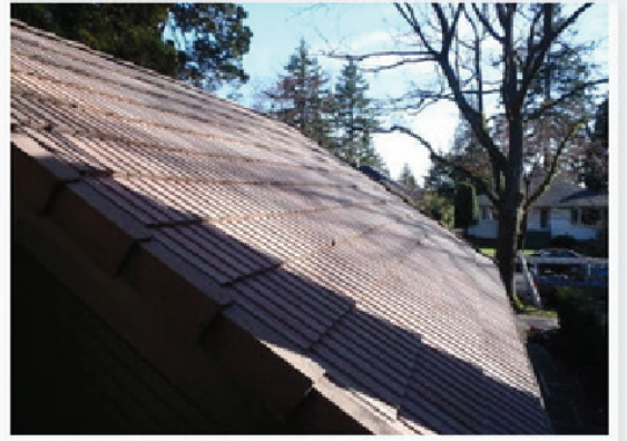
ROOF CLEANING, AFTER
