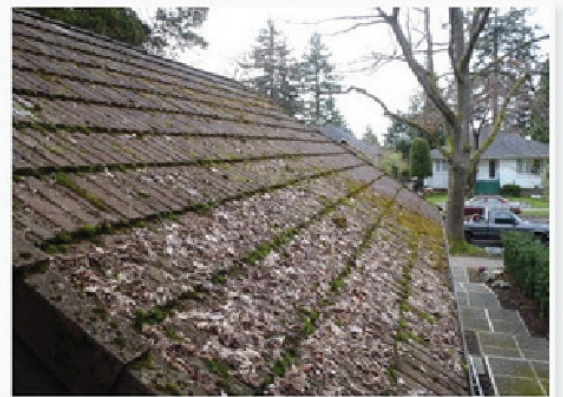
ROOF CLEANING, BEFORE
